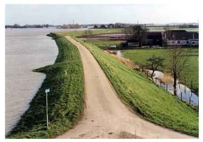
Figure 6-3 Earth levee example from the Netherlands (California Water Blog, 2015)
