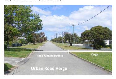
In rural areas, the 'verge' is the portion of land that lies between the top of the back slope of the roadside drain and the adjacent property boundary.
