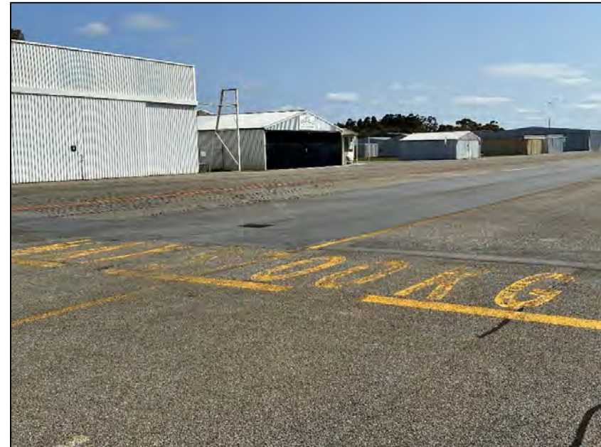
Figure 23 General aviation hangars
