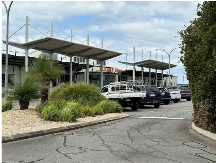
Figure 16 Albany Airport terminal building
