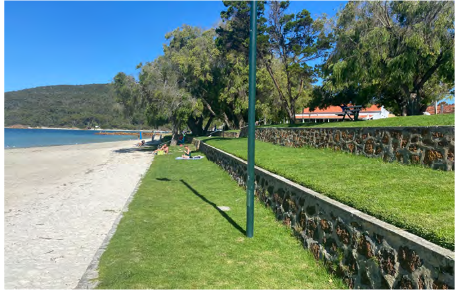
Figure 6 Existing terrace walling (Site photo)
