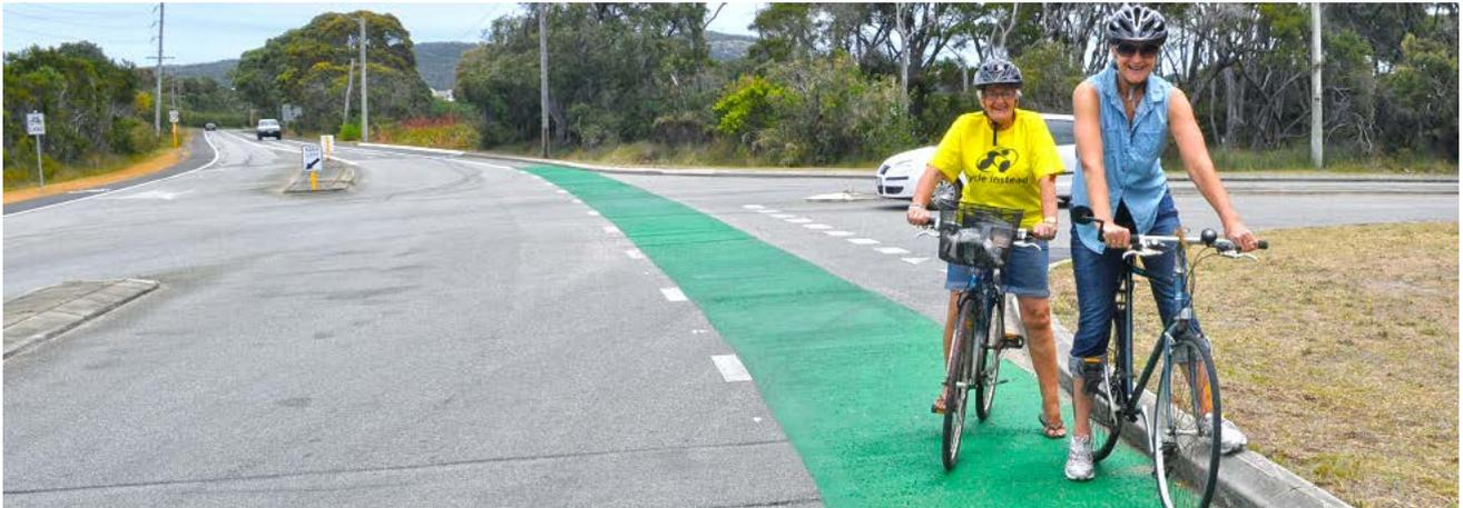
In one of the first initiatives of its kind in regional WA, new bike lanes have been installed between Middleton Beach and Emu Point which include a section of “green treatment” to enhance the visibility of cyclists and increase safety.
