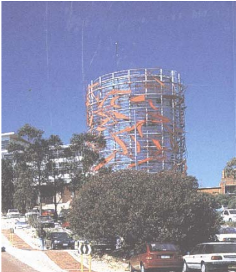
This image shows how a tall functional building element without windows can be creatively treated.
