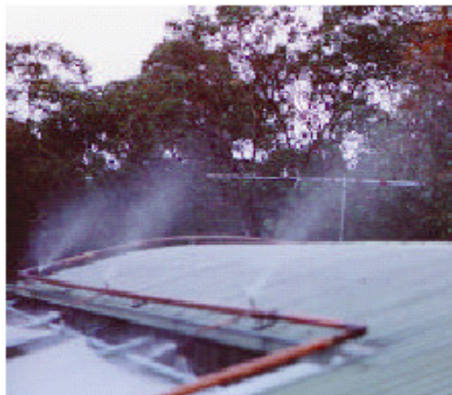
Diagram 1 – Example of roof spray system
