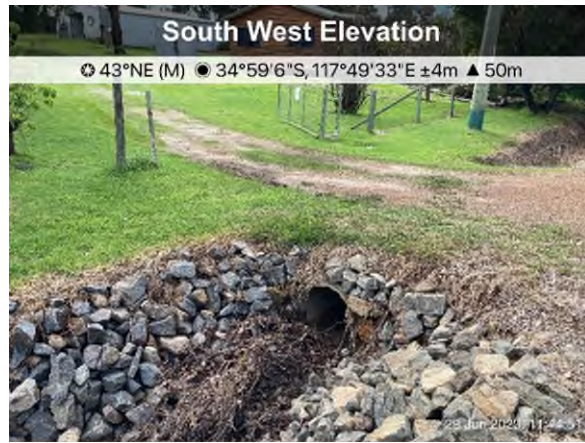
Photo 8: View to the northeast of Lancaster Road roadside swale driveway culvert crossing.
