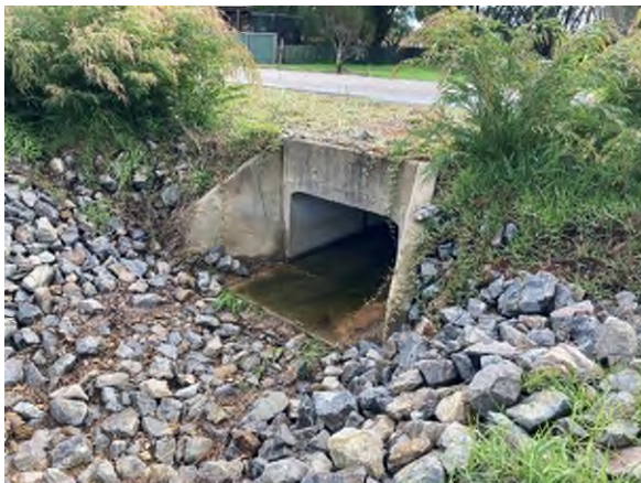
Photo 3: View to the northwest of box culvert (downstream end) under Lancaster Road. Box culvert is 750mm high x 1200mm wide.
