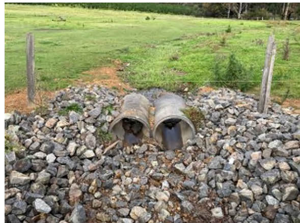
Photo 4: View to the south from Lancaster Road of culverts discharging to creek line within the south of the Subject Site. Culverts are 2 x 750mm diameter.
