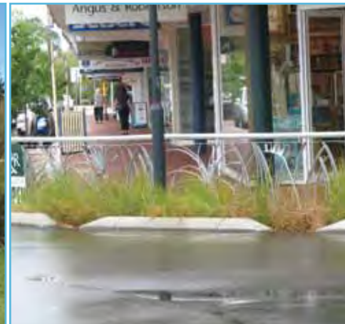
Roadside biofilter retrofit, Busselton CBD
