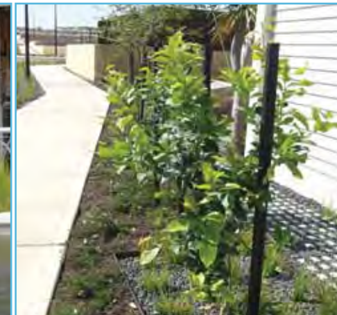
On-lot biofilter, Evermore Heights, Baldivis
