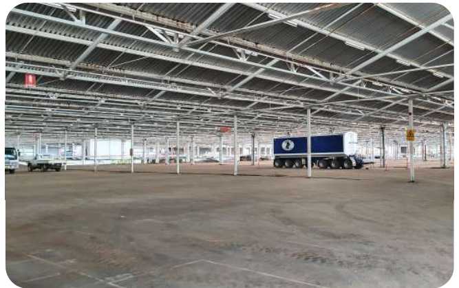
Plate 27 Site image internal view of existing shed (southern) lot 1209
