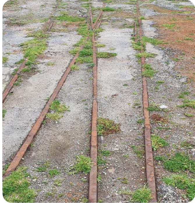
Plate 30 Site image of embedded railway tracks
