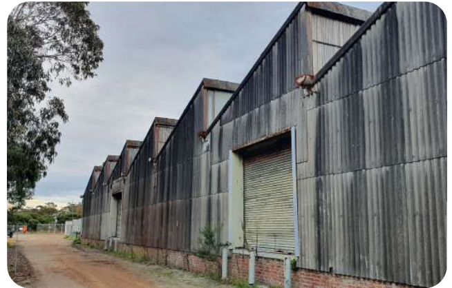
Plate 26 Site image existing Woolstores shed (southern) lot 1209
