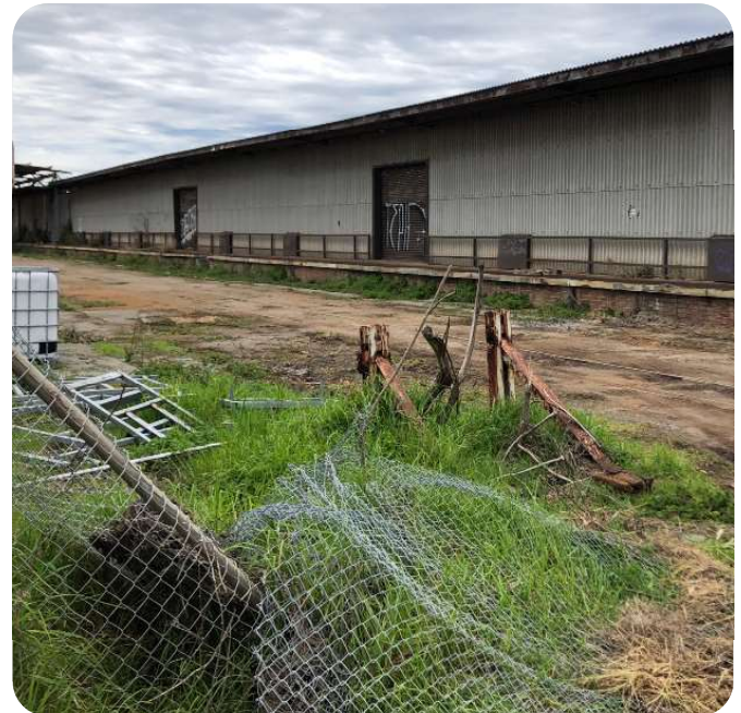
Plate 45 Site Image of current Woolstores Sheds as key visual landmark
