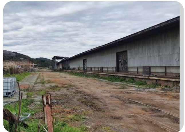
Plate 8 Site Image taken between the two main buildings with gravel access tracks (rail and road).
