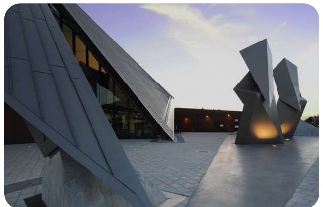
Plate 47 Example of site responsive design, Albany Entertainment Centre by Cox Architects
