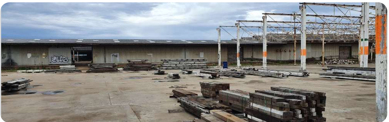
Plate 28 Site image looking towards northern shed with partial demolition underway
