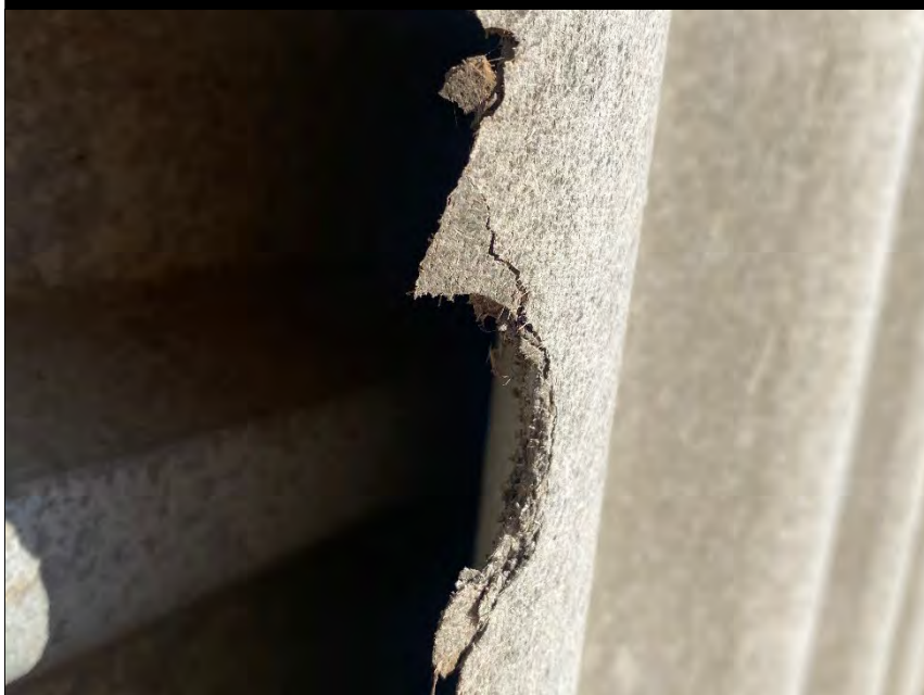
POTENTIAL BROKEN ACM FENCING
