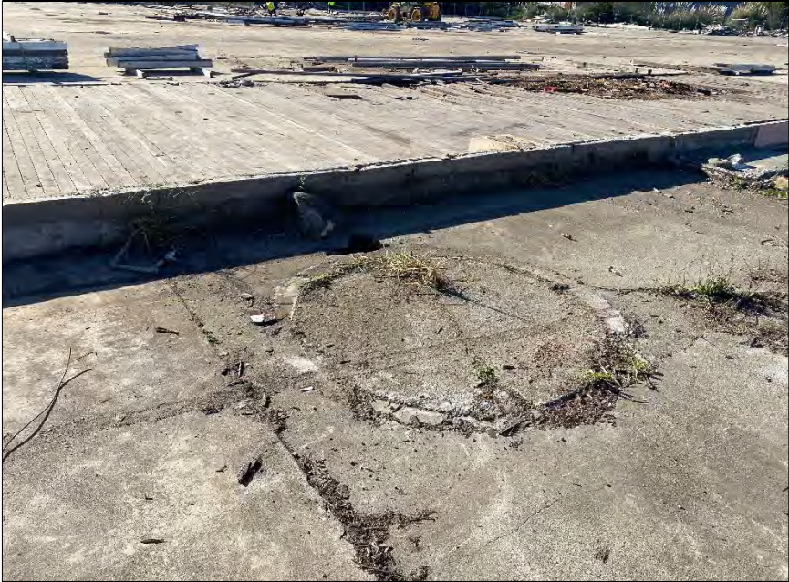
OUTDOOR LAYDOWN AREA / CRACKED BITUMEN
