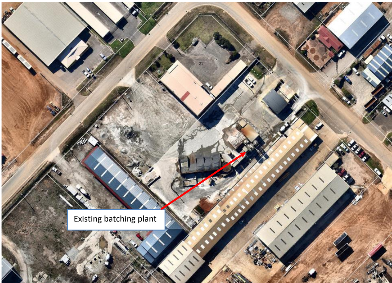
Figure 4: Existing Batching Plant location
