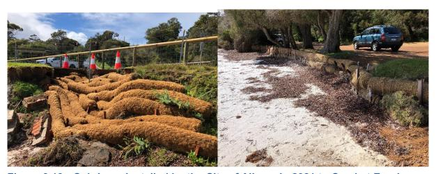
Figure 3.13 Coir Logs Installed by the City of Albany in 2021 to Combat Erosion
