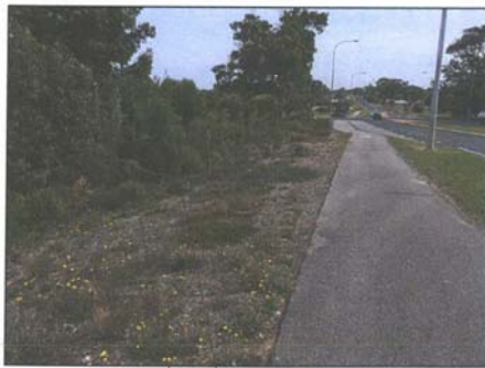
EXISTING GRASS COVER TO BE REMOVED AND RE-PAVED. THIN OUT LARGE CLUSTERS OF SMALL SHRUBS.
