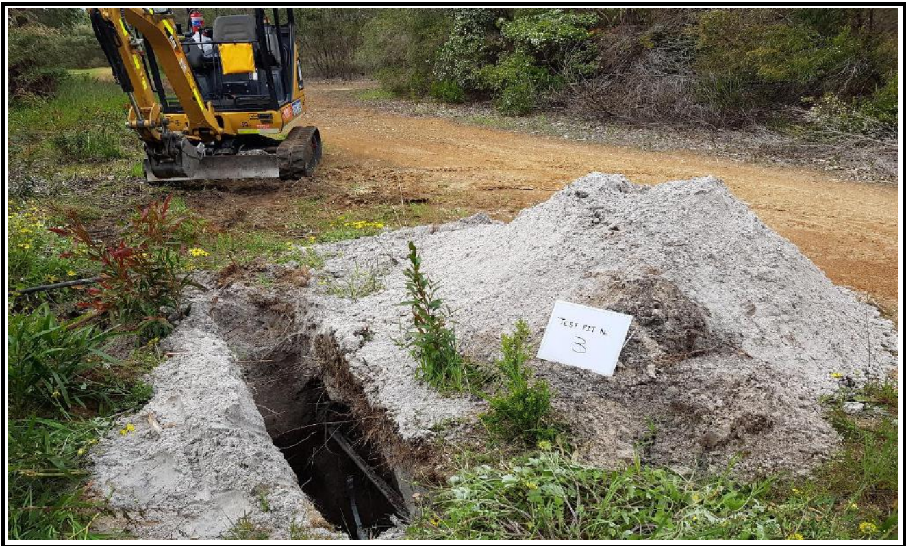
Test Pit No. 3 Spoil
