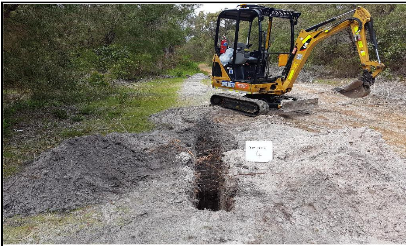
Test Pit No. 4 Spoil
