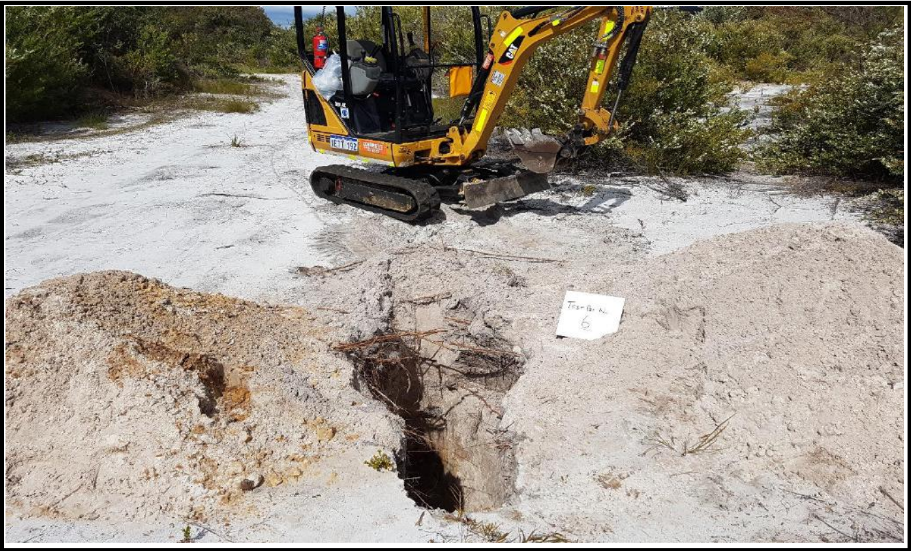
Test Pit No. 6 Spoil
