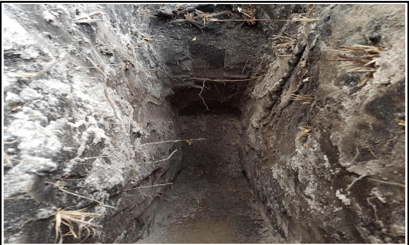
Test Pit No. 2 Excavation
