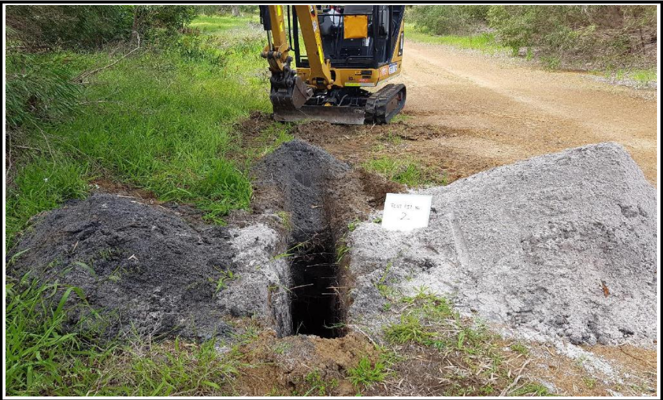
Test Pit No. 2 Spoil
