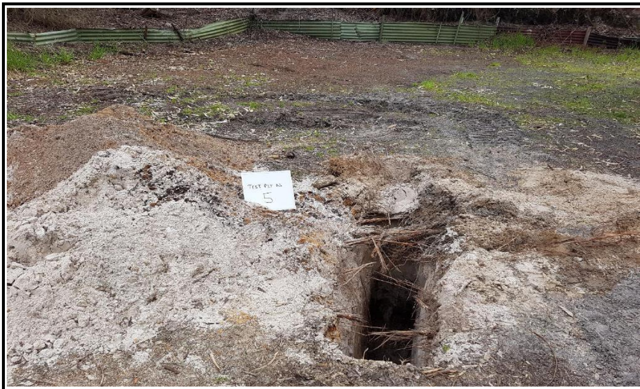
Test Pit No. 5 Spoil
