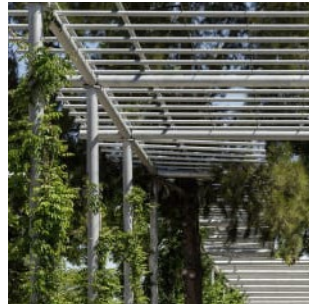
Balcony trellis - galvanised metal
