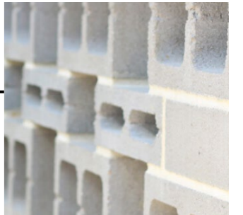
Apartment fences and screening - raw limestone finish blockwork walls
