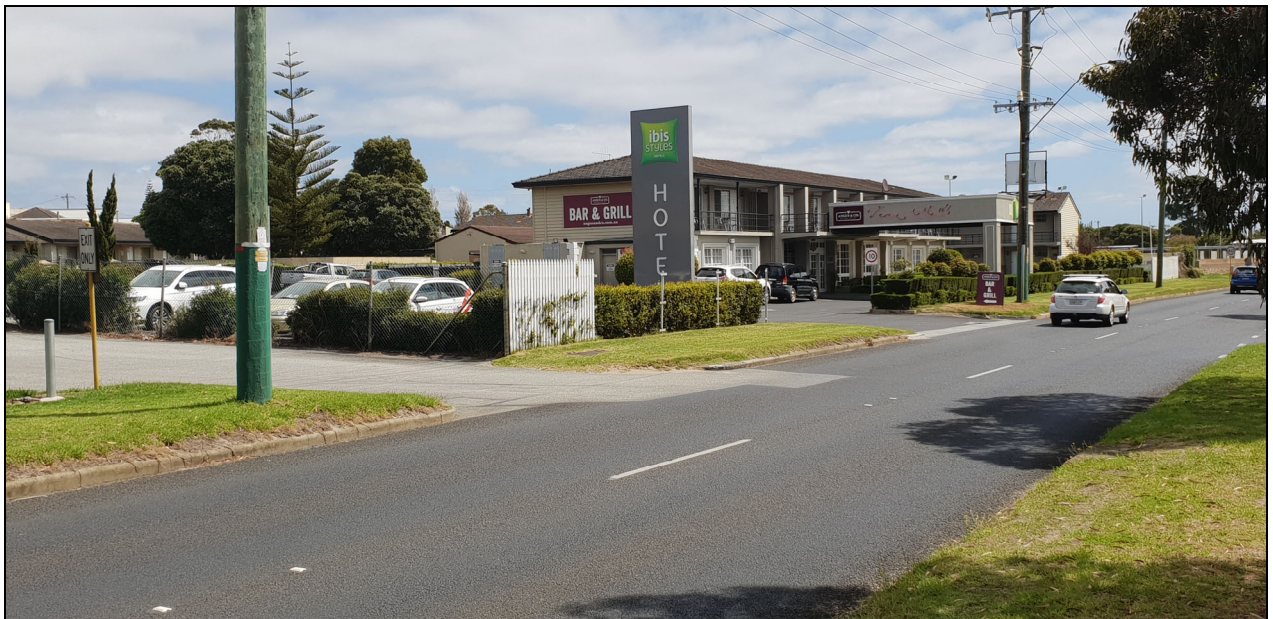
Photo 4: View of exit on to Albany Highway and adjoining Ibis Styles Hotel
