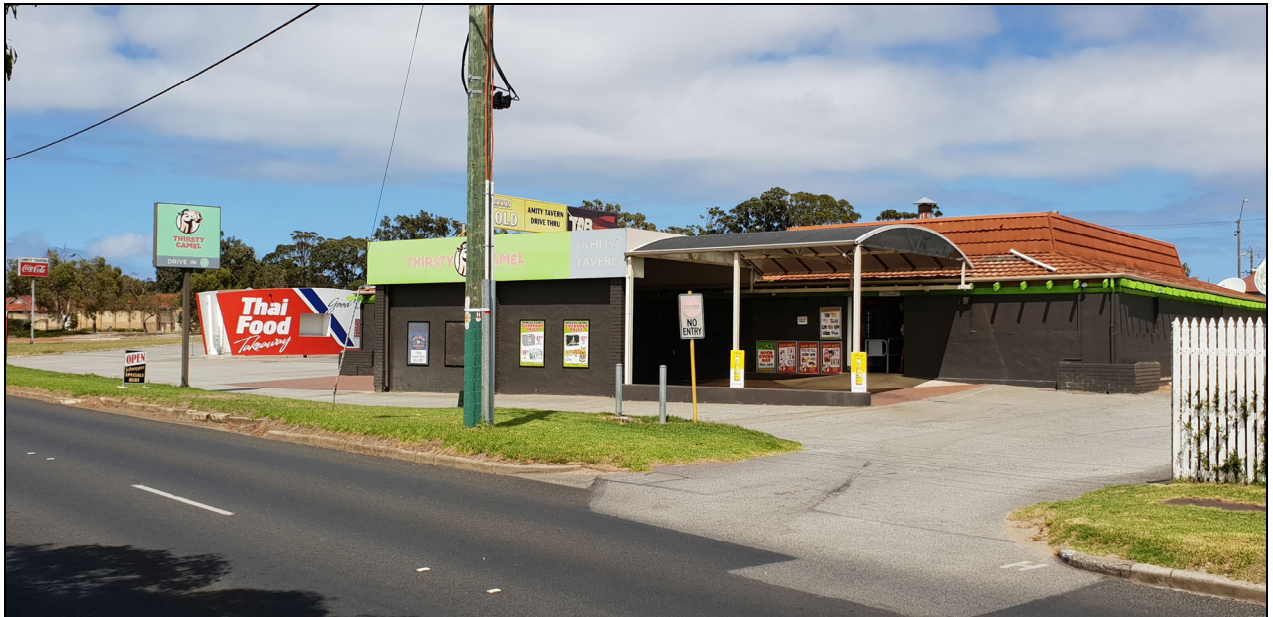
Photo 3: View from north showing Amity Tavern and drive through bottle shop.
