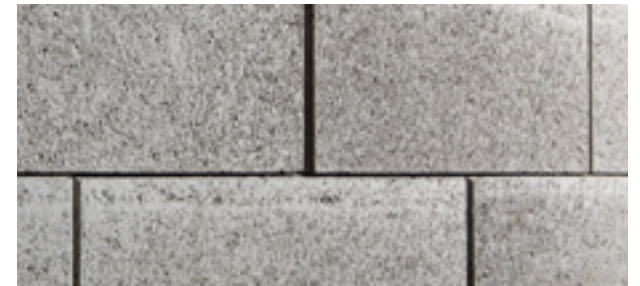
9. Block Work Walling
