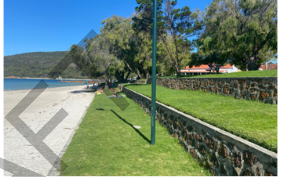
Figure 6 Existing terrace walling (Site photo)
