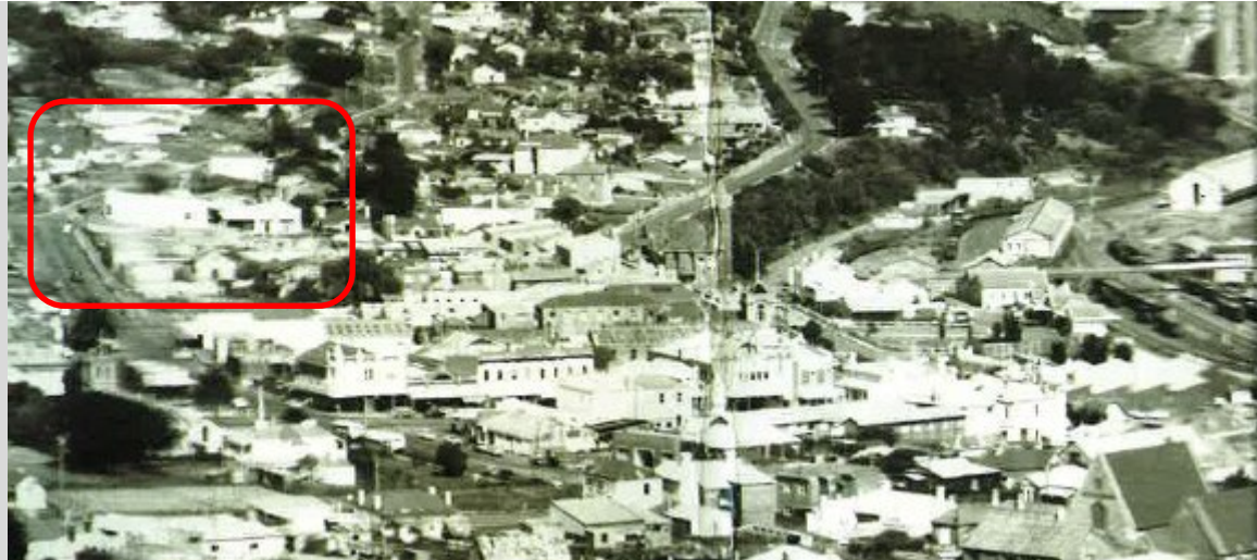
Photo 12. Detail view of archival photo from c1958 showing subject buildings highlighted. The single two-bay façade of the commercial building is evident, but not the subsequent extension, although there appears to be a covered drive-thru roof in this location. Note only two windows evident on the corner building.
