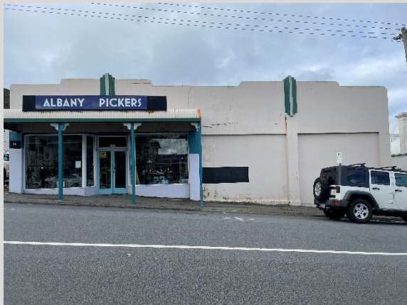
Photo 9. Spencer St (west elevation)
