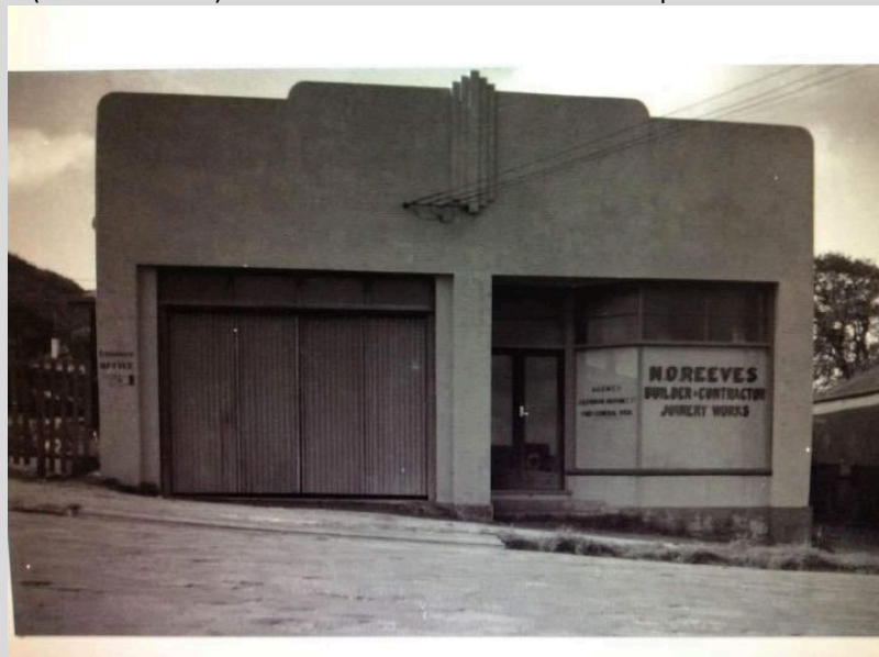
Photo 11. Undated archival photograph of Reeves Hardware building, sourced from Lost Albany facebook page, 2022, likely dates from early 1950s. Note the façade only comprised two bays, not four. On the basis of the adjoining residence (to the south), this would suggest that the building was later extended northward towards the corner building, most likely in the 1950s.
