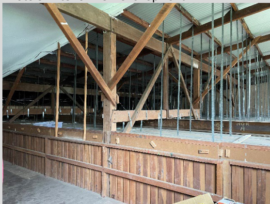
Photo 7. Interior view of exposed roof structure
