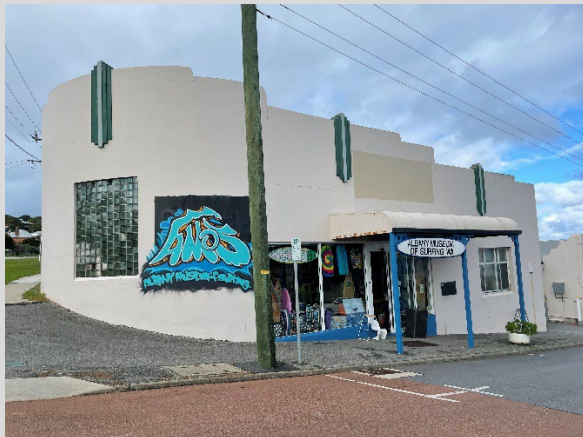
Photo 1. Spencer St (west) elevation
