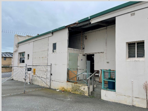
Photo 4. South elevation with loading bay
