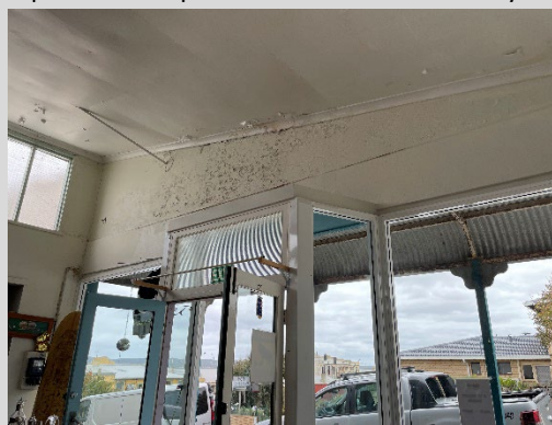
Photo 16. Interior view of shopfront
