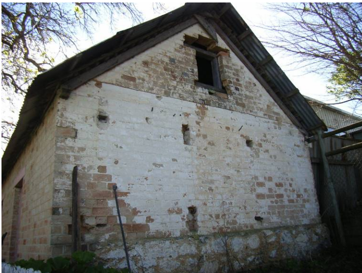
East elevation [H Munt 2008]
