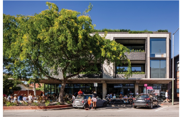
Design Guide – adaptable ground floor level, residential above with opportunities to convert ground level to commercial space.
