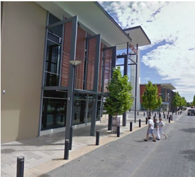
Design Guide – nil boundary setback, and building floor levels consistent with adjacent verge level, building height and roof together with design of building provide relationship to the street.
