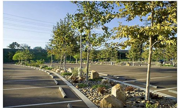
Design Guide – tree planting in extensive car park area, water sensitive urban design principles for stormwater infiltration, vehicle stop guards to protect trees and cars.
