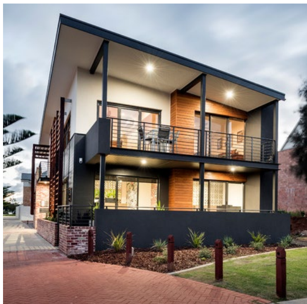
Design Guide – residential development designed to provide surveillance of the street, articulation and interest.
