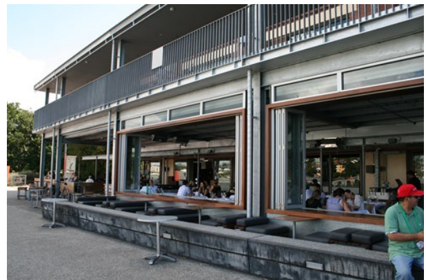
Design guide – balconies and large openings in buildings to promote surveillance and activation.
