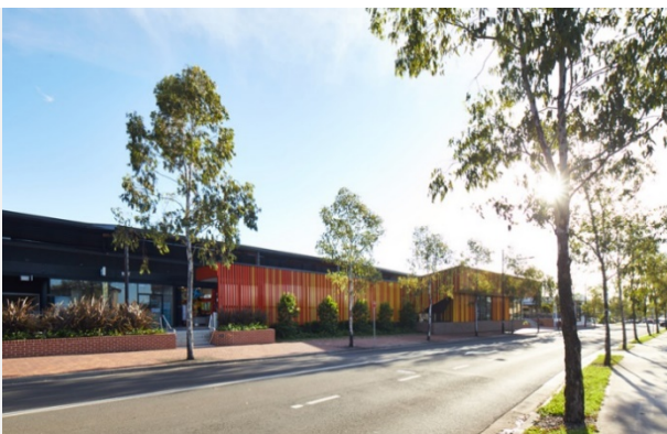
Design Guide – Ground level commercial frontage, providing awning and glazing, providing a connection to the street.
