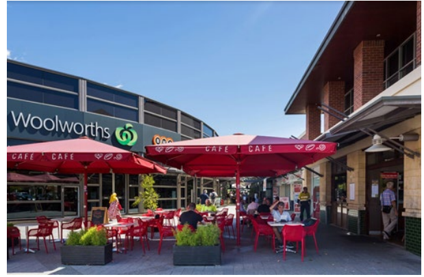
Design Guide – utilisation of space adjacent to mixed use development and supermarket for alfresco seating and food and beverage opportunities.
