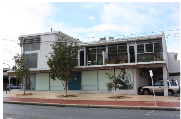
Design Guide – residential incorporating adaptable ground-level frontages to the street, which can be converted in future.
