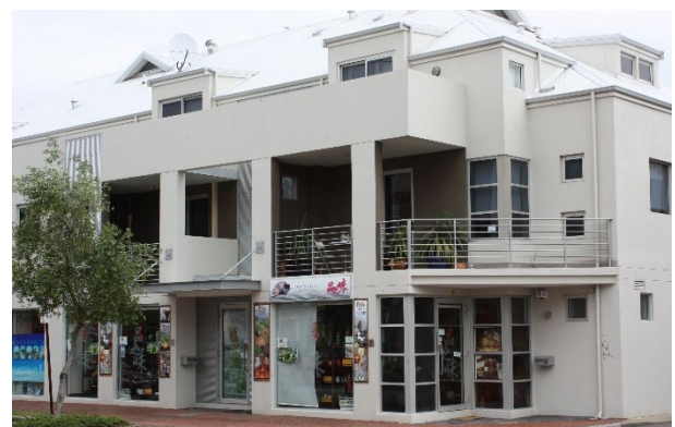
Design Guide – residential component of buildings incorporating large windows, balconies and living spaces overlooking the street / public open space; adaptable frontage at ground level.
