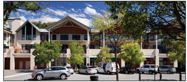
Design Guide – adaptable ground floor level, residential above with major openings and balconies overlooking the street.
