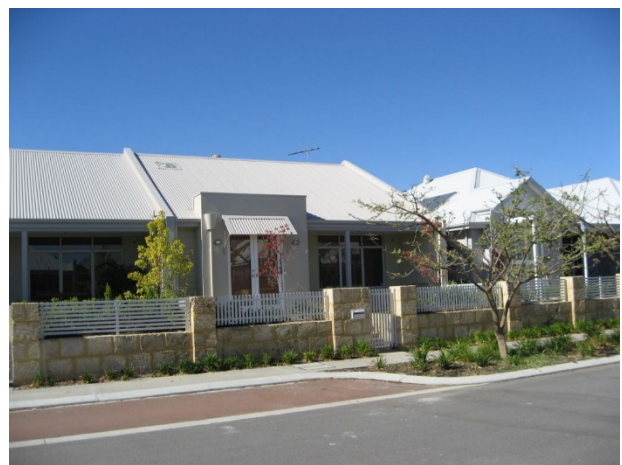
Design Guide – dwellings with low fencing and orientation to street, street upgrades providing visitor parking and street trees.
