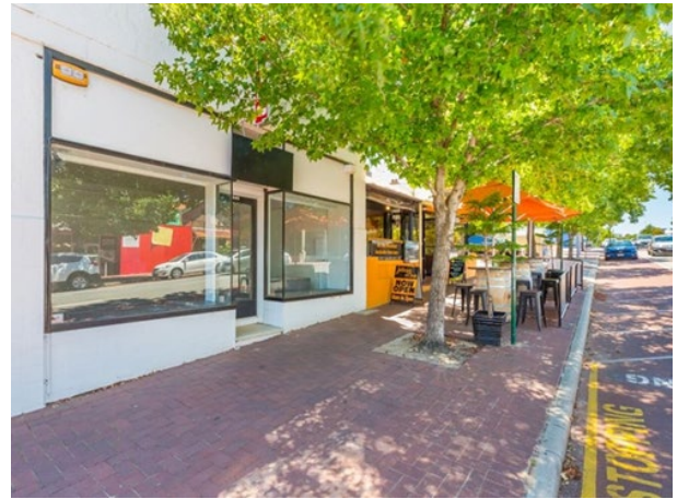
Design Guide – legible entry and glazing, nil boundary to a main street, presenting an active street frontage.
