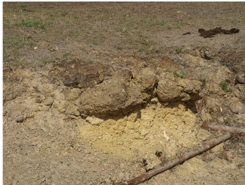
16. Exposed soil profile – edge of dam at site 19 showing subsoil clay beneath laterite boulder layer within upland terrain land unit U2.
