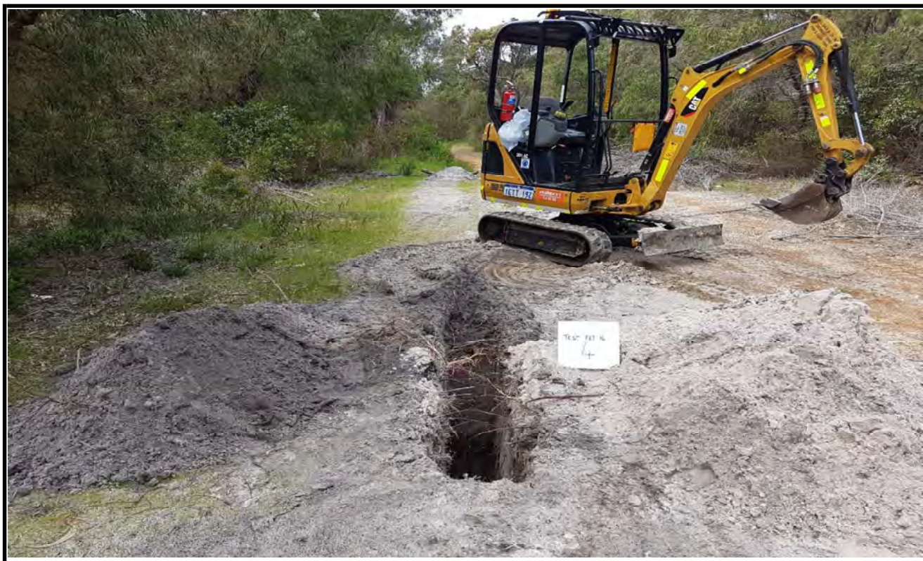
Test Pit No. 4 Spoil
