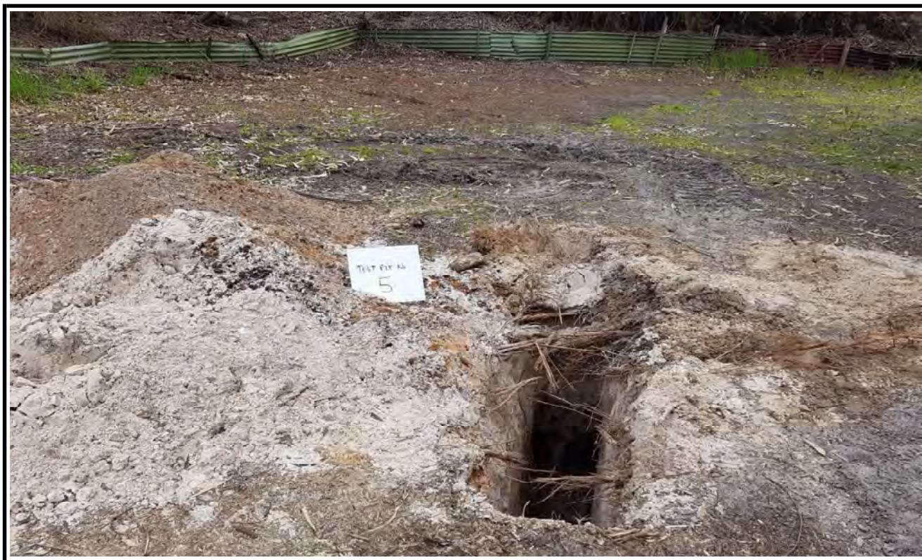
Test Pit No. 5 Spoil
