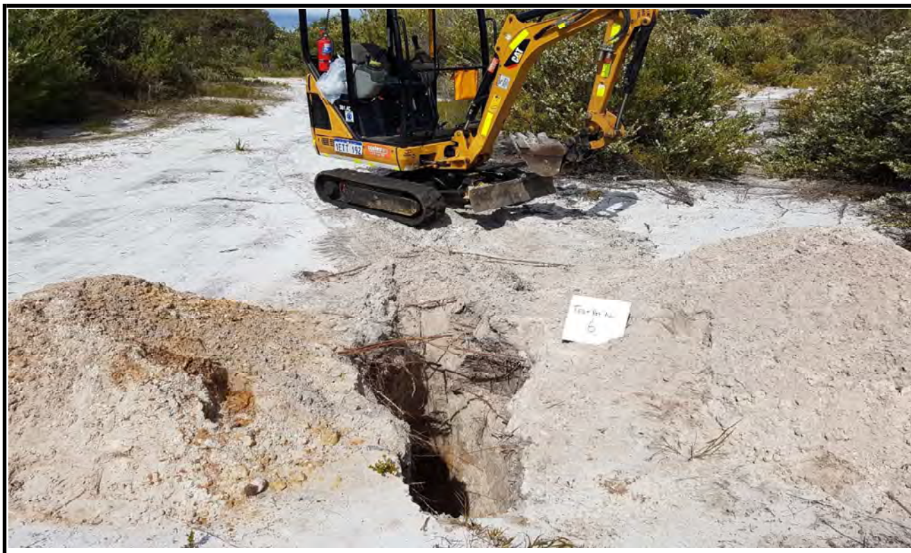
Test Pit No. 6 Spoil
