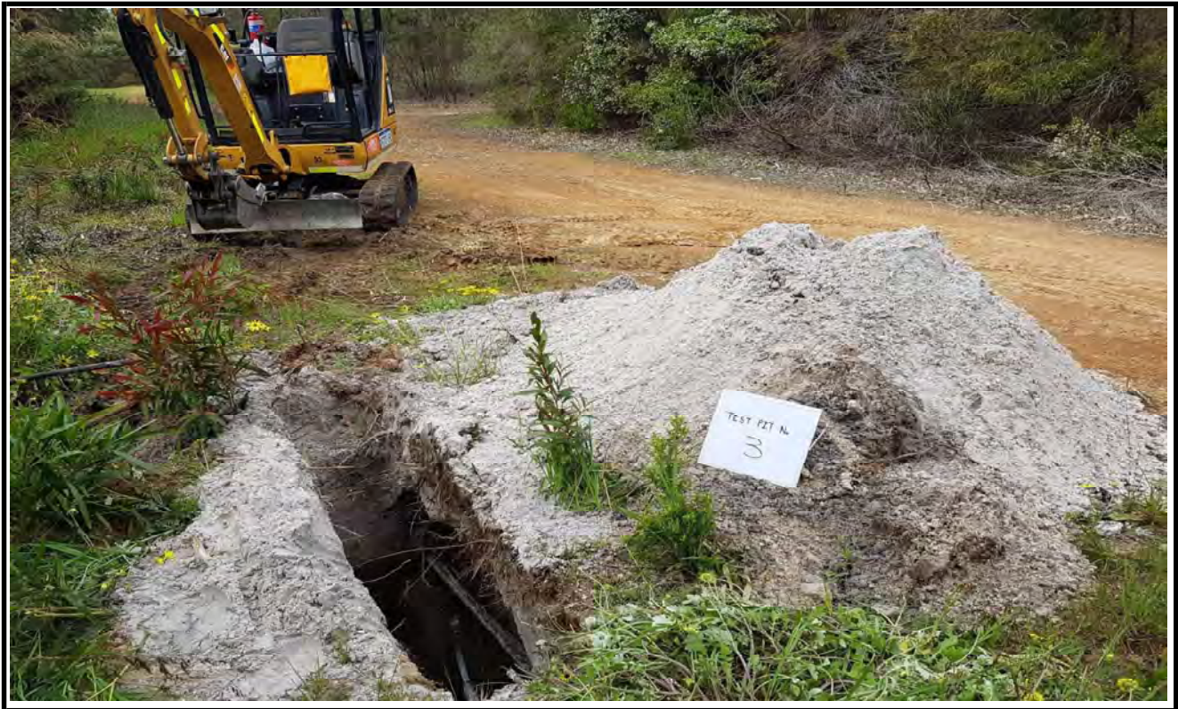
Test Pit No. 3 Spoil
