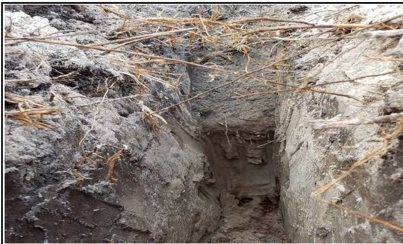
Test Pit No. 4 Excavation
