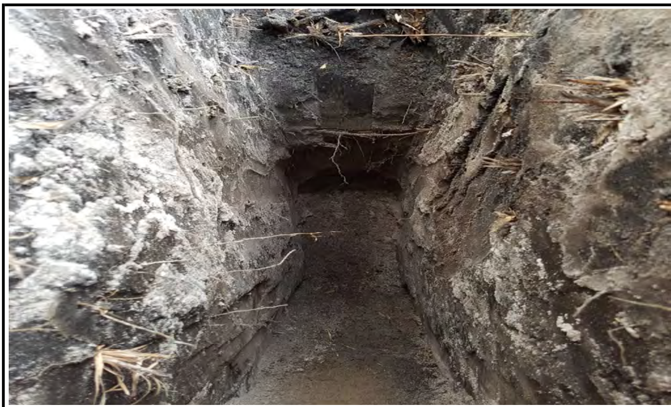
Test Pit No. 2 Excavation
