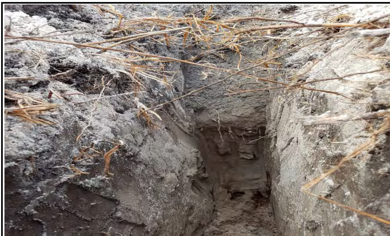
Test Pit No. 4 Excavation
