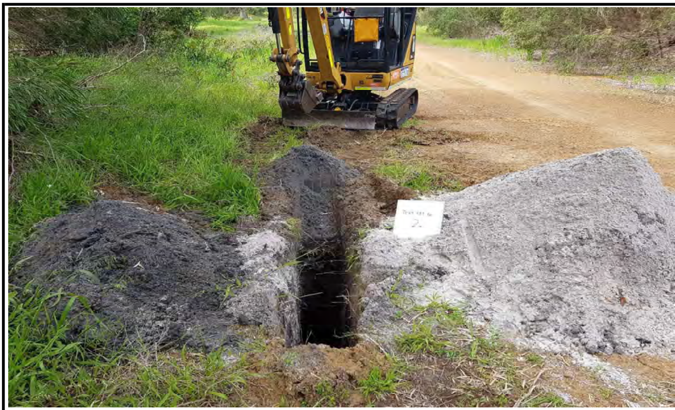
Test Pit No. 2 Spoil
