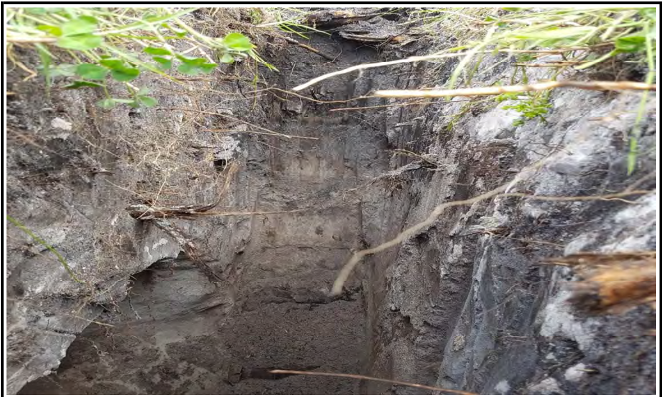
Test Pit No. 1 Excavation
