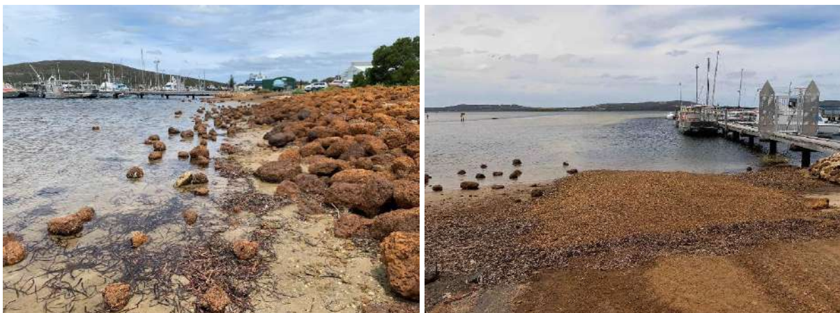
Figure 2.2 Existing Seawall (Left) & Gravel Ramp (Right)
