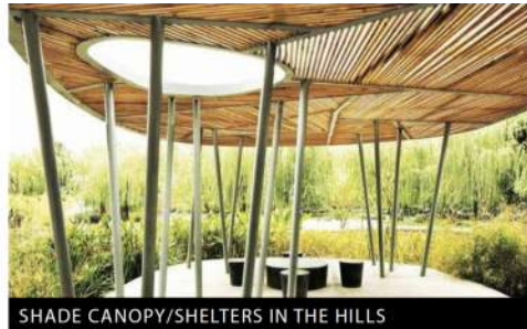
SHADE CANOPY/SHELTERS IN THE HILLS
