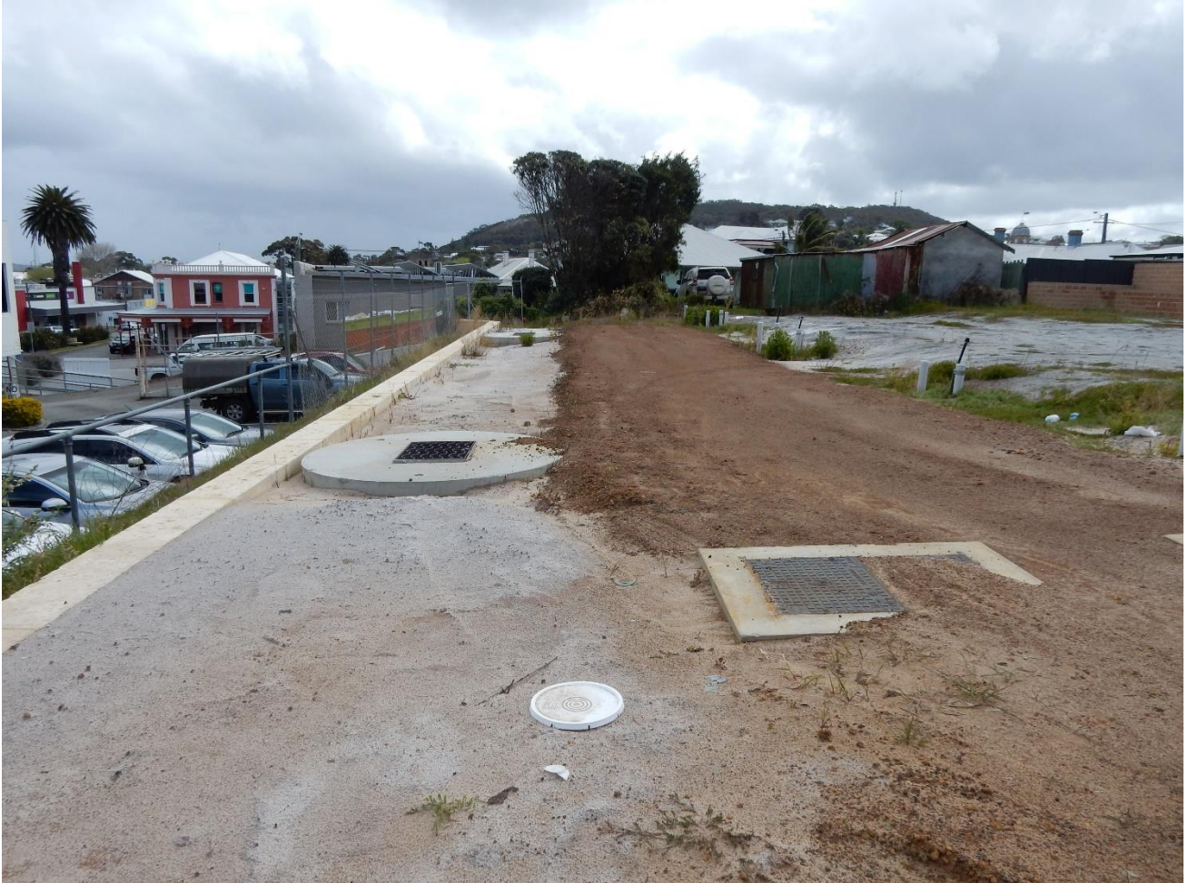
Figure 1: ROW shown from eastern boundary looking west (photo taken 6/10/2022)
