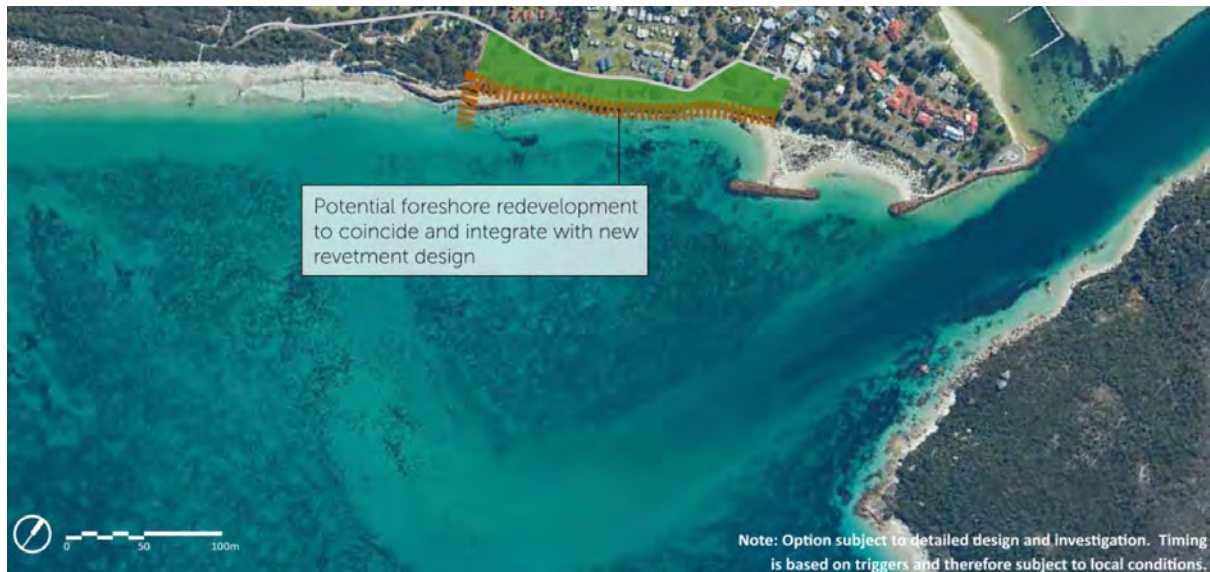
Figure 6: MU4 Foreshore Reserve CHRMAP recommendation19: Foreshore Reserve - Revetment be upgraded along with redevelopment of Foreshore park and removal of sandbag revetment (source: Aurora, 2019).
