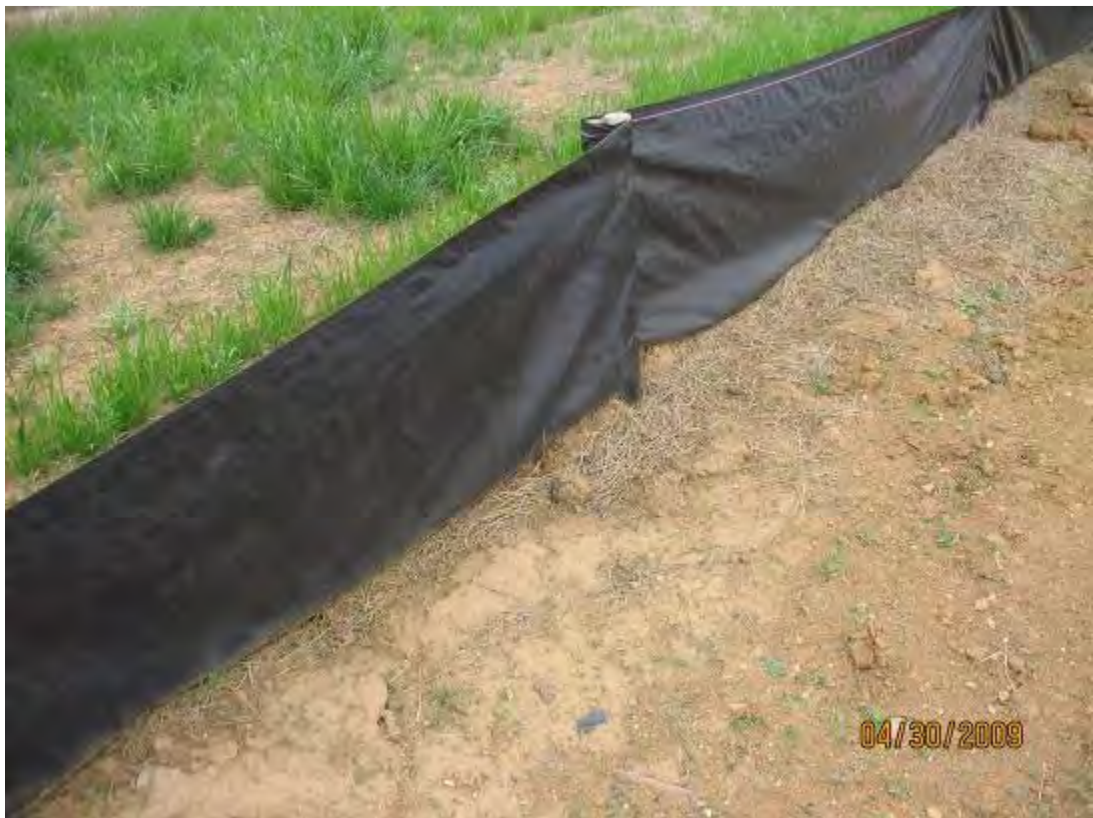
Silt trapping fence
