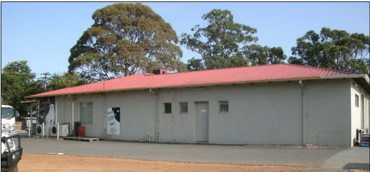
Photograph 5 – Existing retail building façade, southern elevation.
