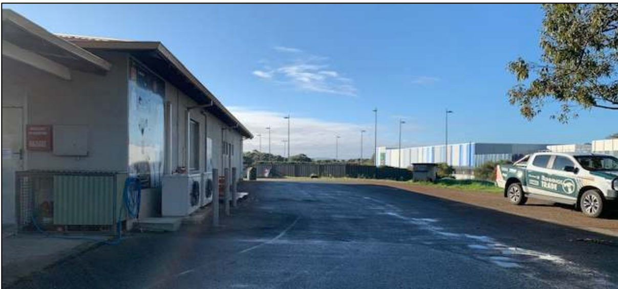
Photograph 6 – Rear of subject site showing informal parking.
