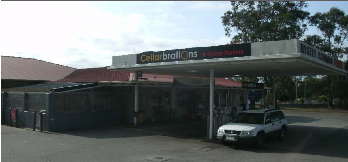
Photograph 1 – Retail building and refuelling facilities, viewed from the north.
