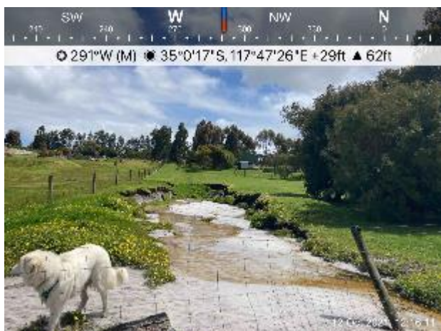
Photo 11: View to the west northwest of eroded drainage easement to the west of eastern corner of Subject Site. Easement discharging runoff and sediment into the Subject Site.
