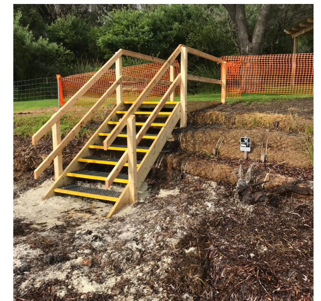
Image 17 Stair access July 2022
