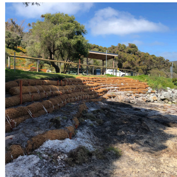
Image 16 Coir log erosion control November 2021
