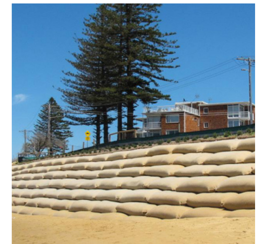
Geotextile sand containers
