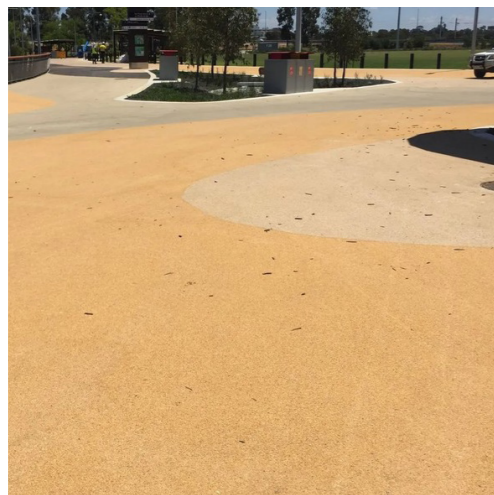
Coloured treatment to asphalt paving
