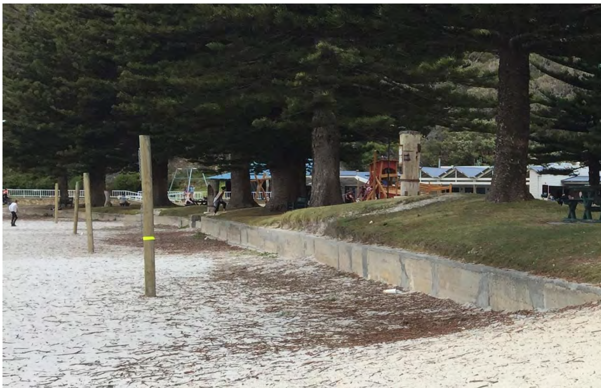
Figure 6.3 Existing Retaining Wall
