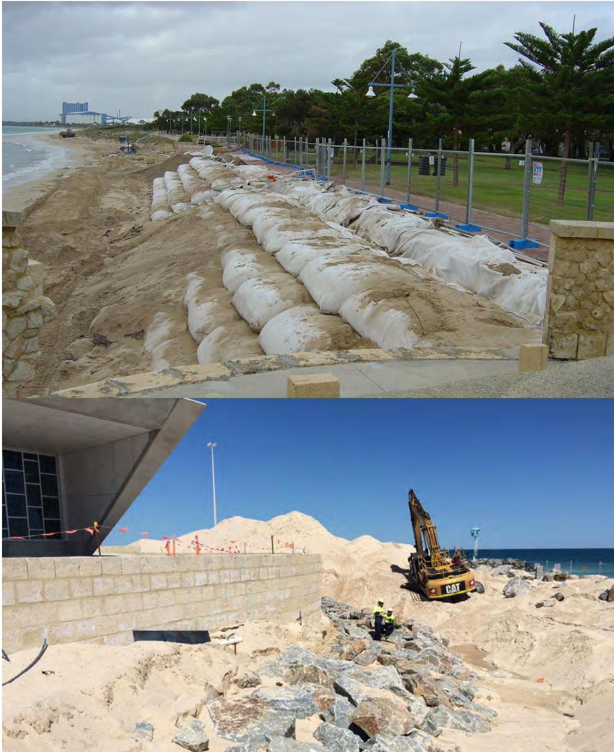
Figure 6.5 Example of a GSC Seawall (Top) and a Rock Seawall (Bottom)
