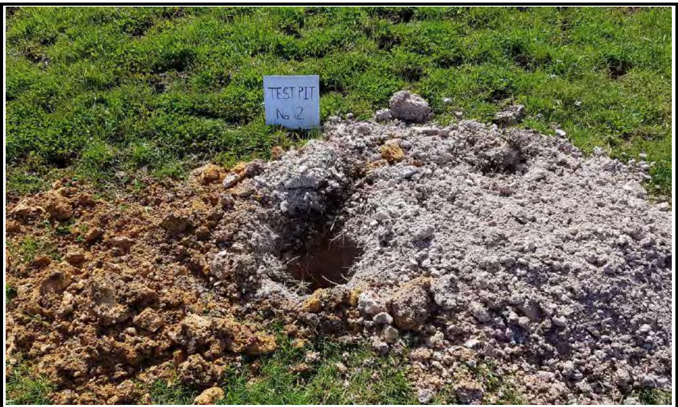
Test Pit No. 2 Spoil
