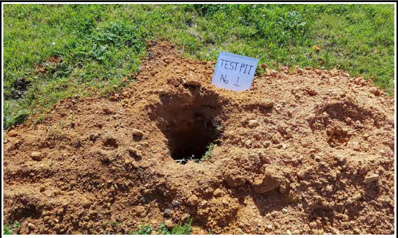
Test Pit No. 1 Spoil
