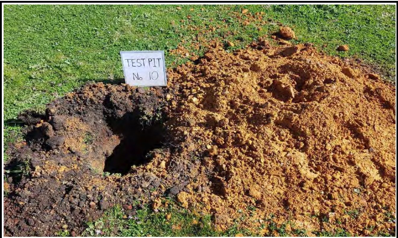
Test Pit No. 10 Spoil
