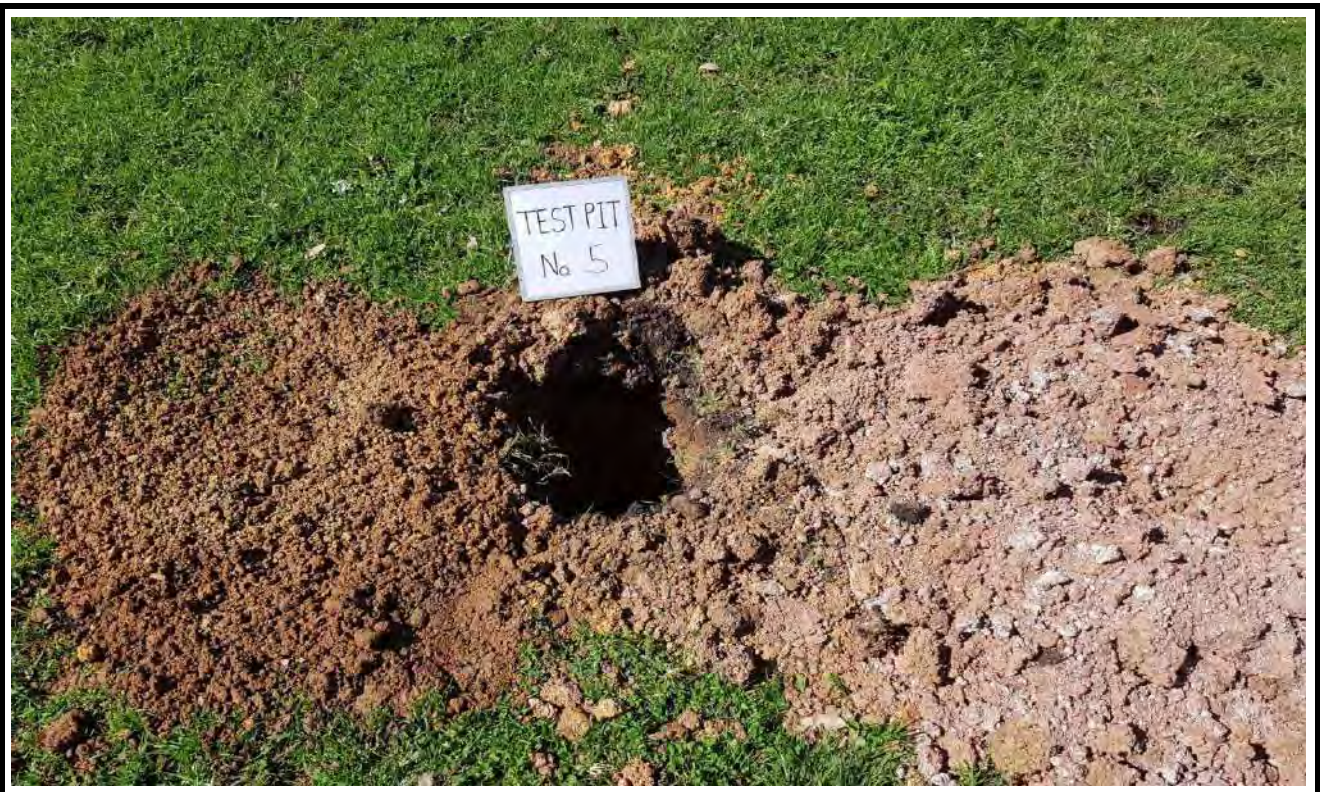
Test Pit No. 5 Spoil
