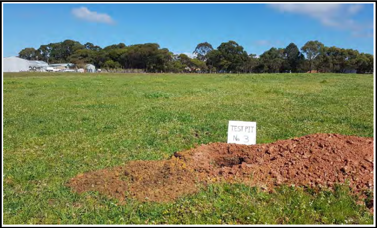
Test Pit No. 3 Excavation
