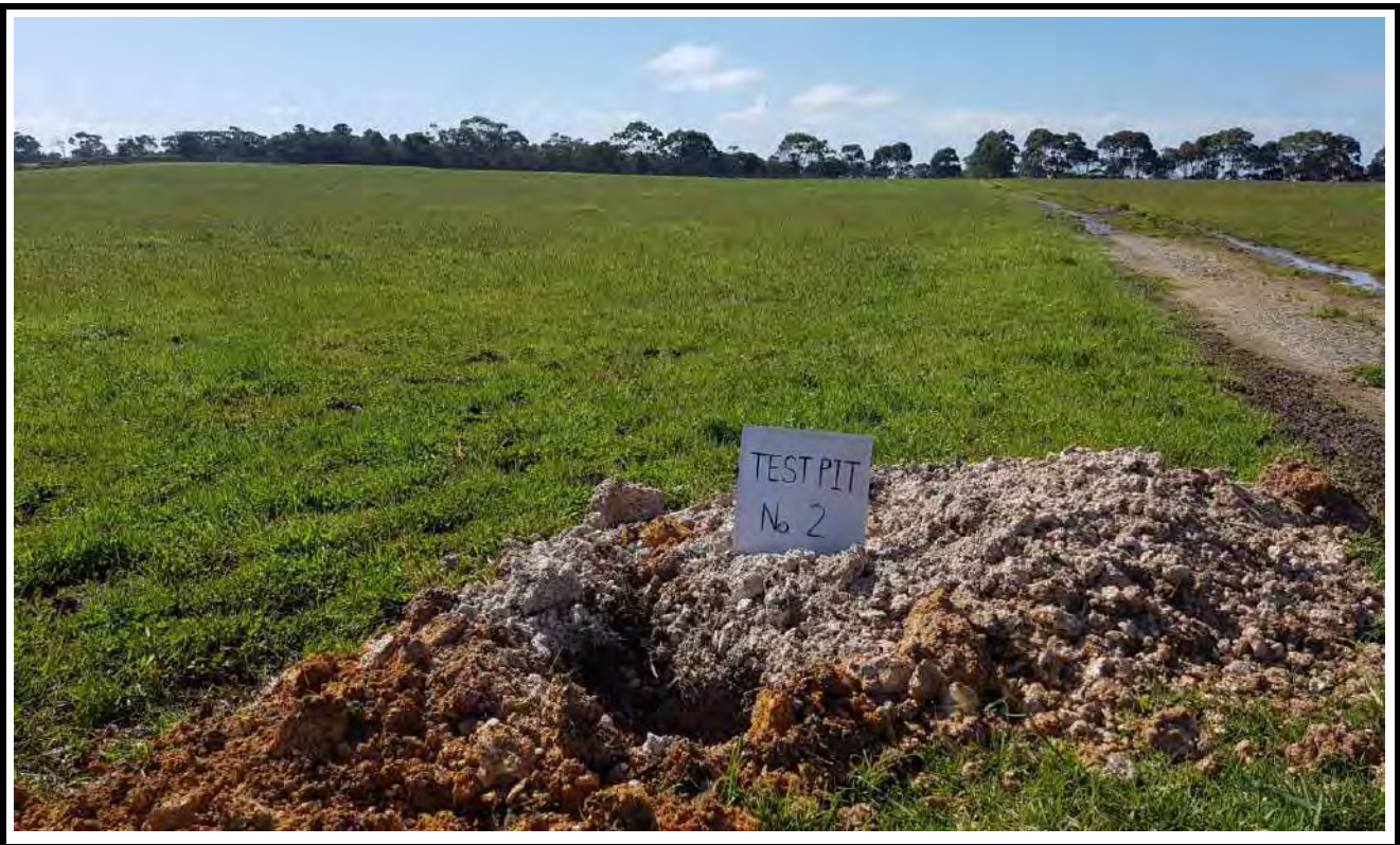
Test Pit No. 2 Excavation
