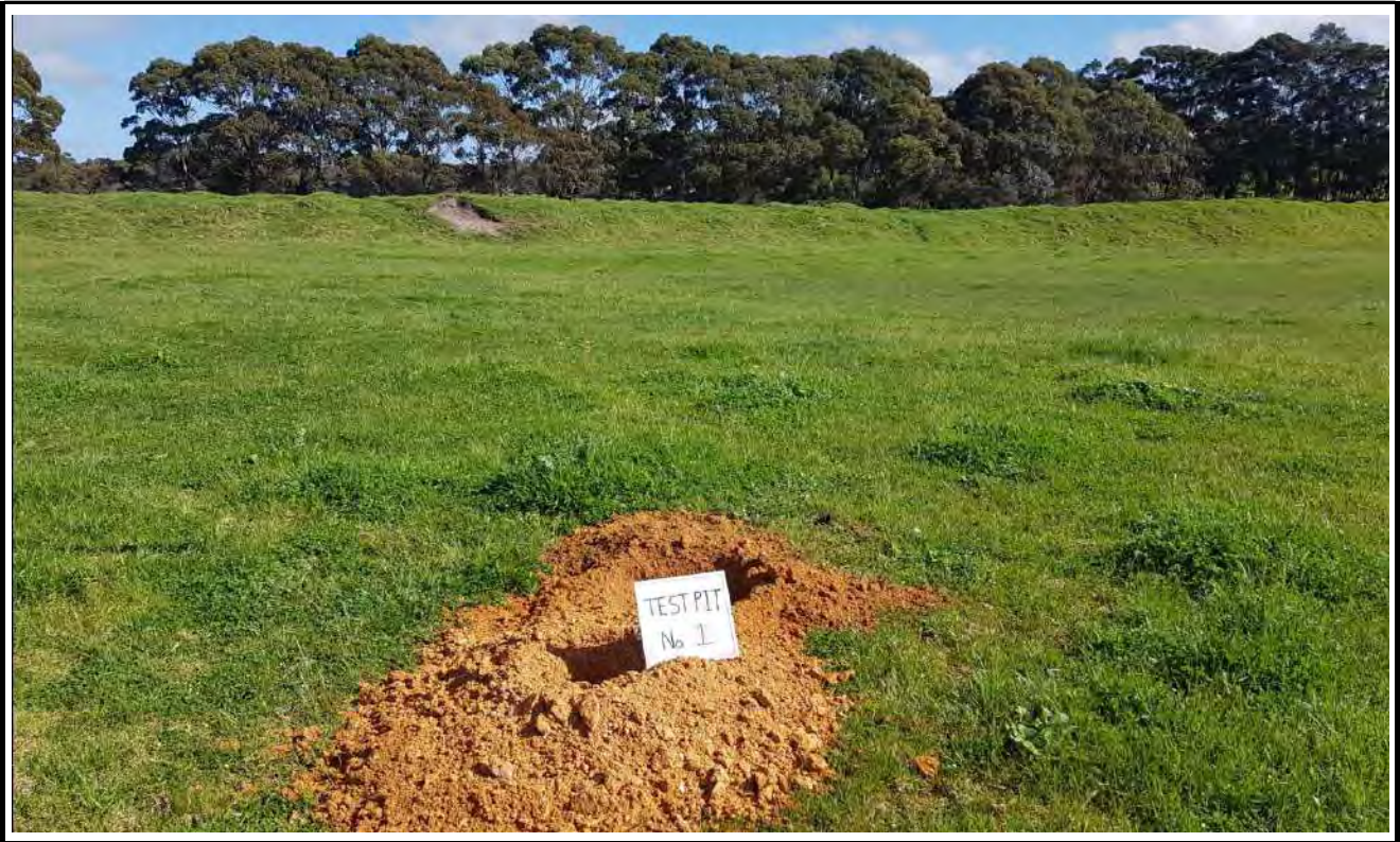
Test Pit No. 1 Excavation
