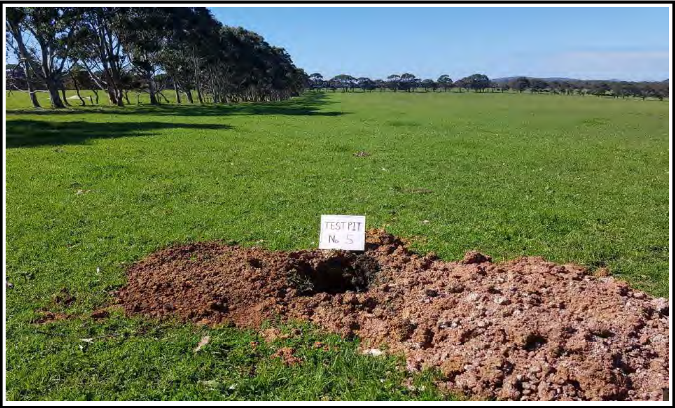
Test Pit No. 5 Excavation
