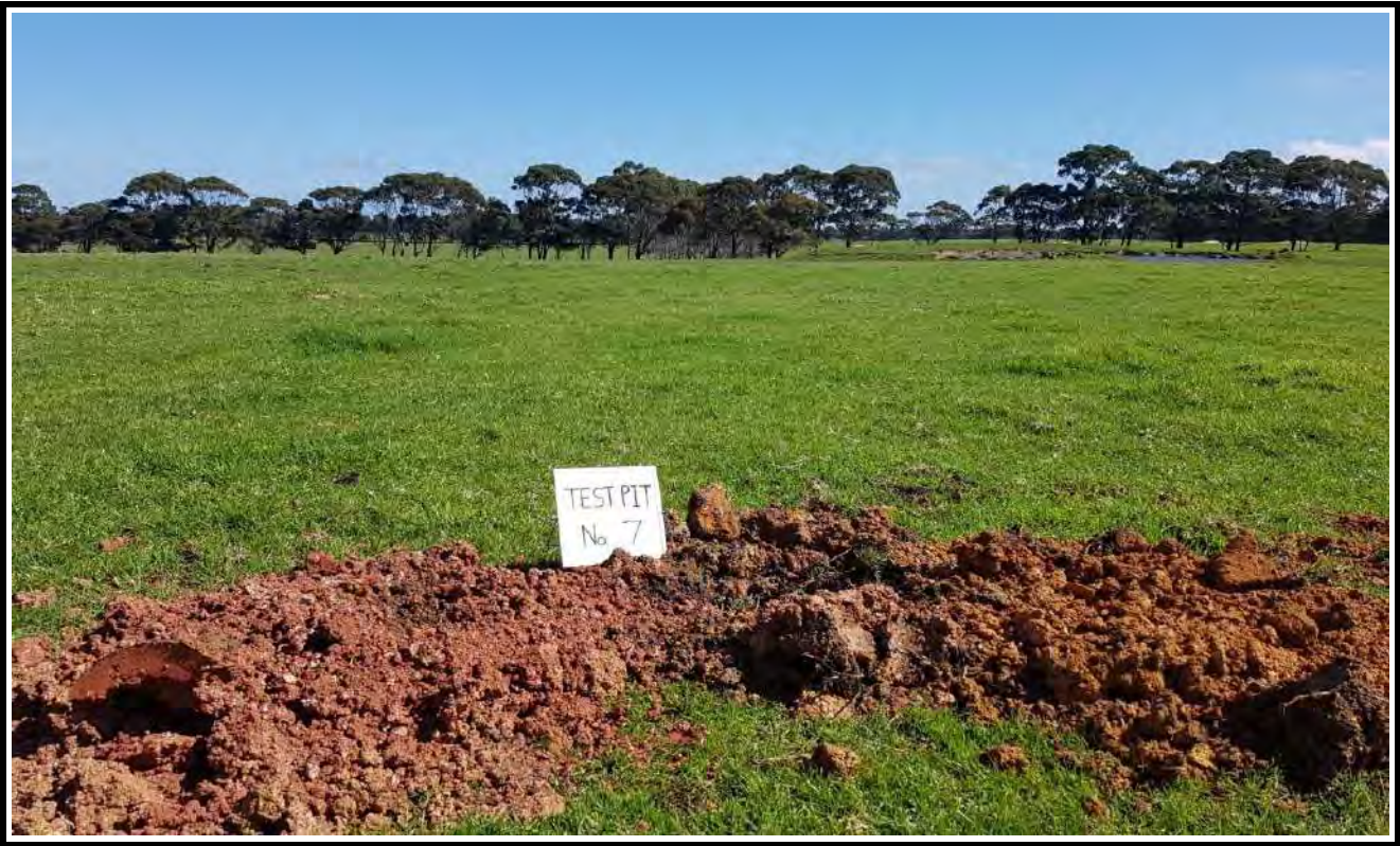
Test Pit No. 7 Excavation
