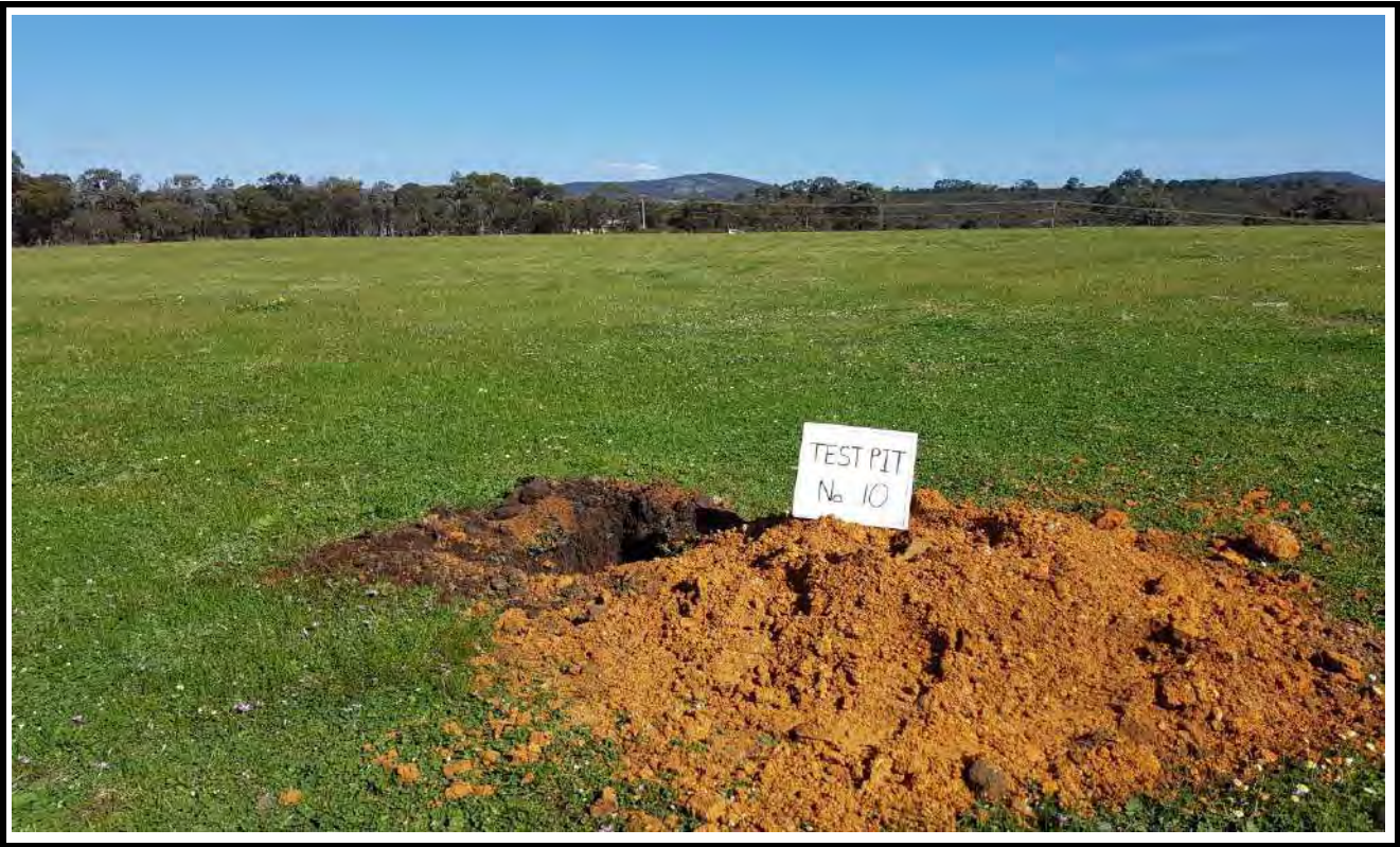
Test Pit No. 10 Excavation
