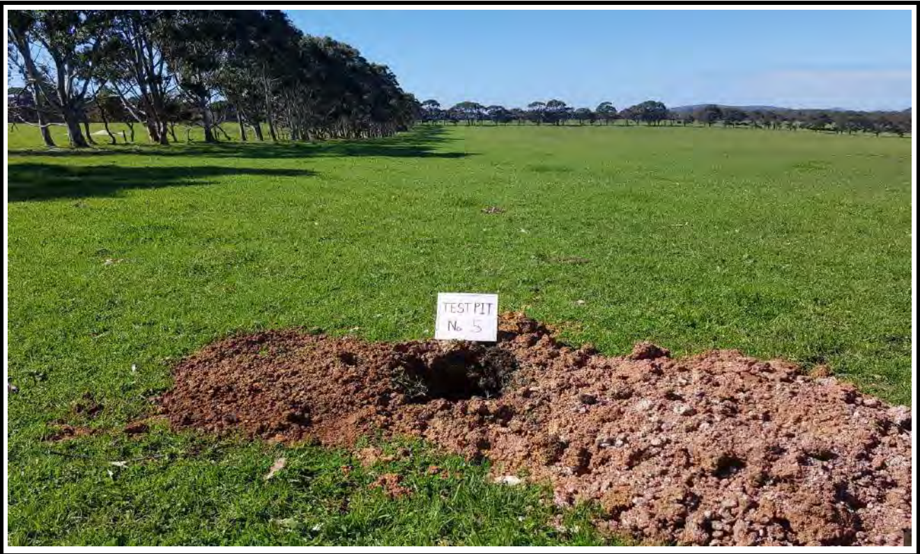
Test Pit No. 5 Excavation
