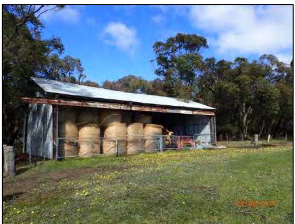
Photograph 3 – View of hay and machinery shed located in the north of Lot 521 Mercer Road.
