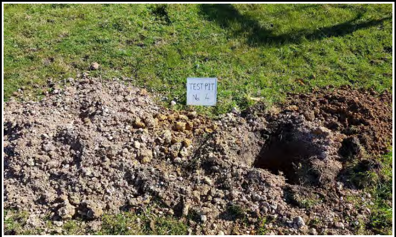
Test Pit No. 4 Spoil
