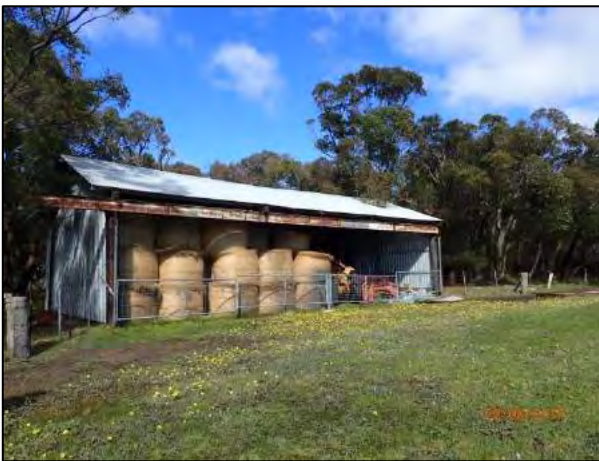
Photograph 3 – View of hay and machinery shed located in the north of Lot 521 Mercer Road.
