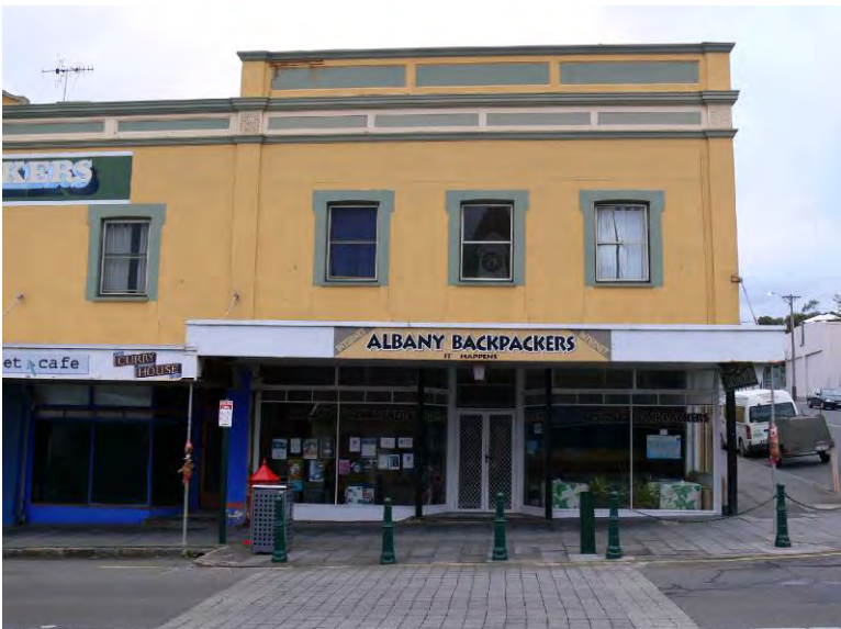
Note former verandah and colour scheme [Heritage Today 2000]
