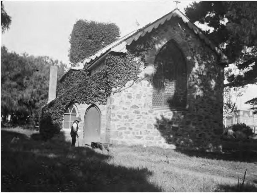
The Church – west elevation (rear), c1915 [SLWA b4380948]
