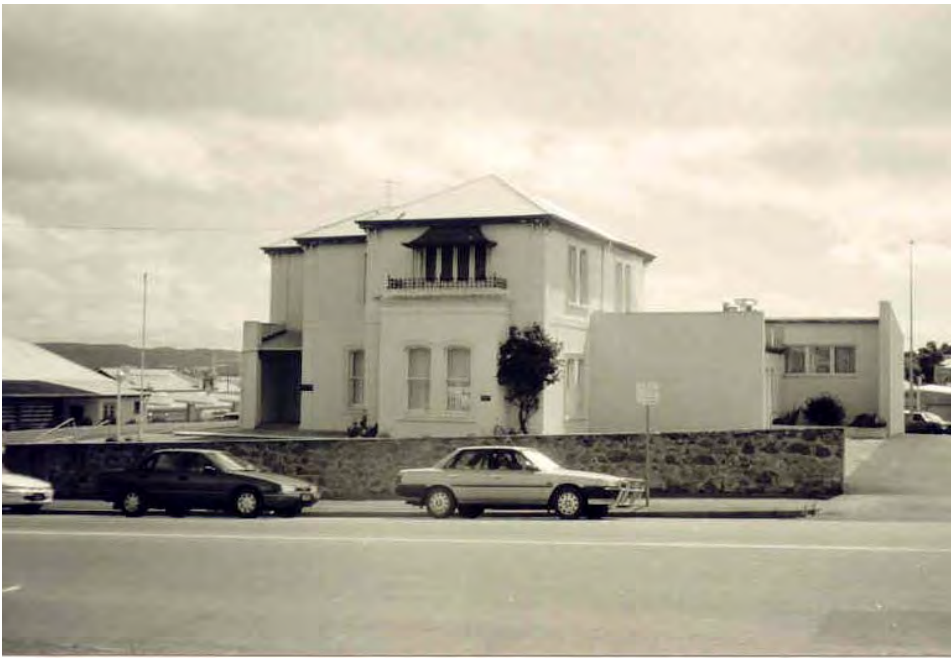
A view of the Albany Club showing the 1960's/1970s extension to the north [Heritage Today 2000]
