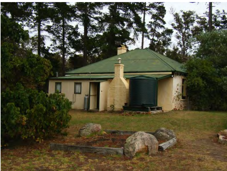
Rear elevation [H Munt 2009]
