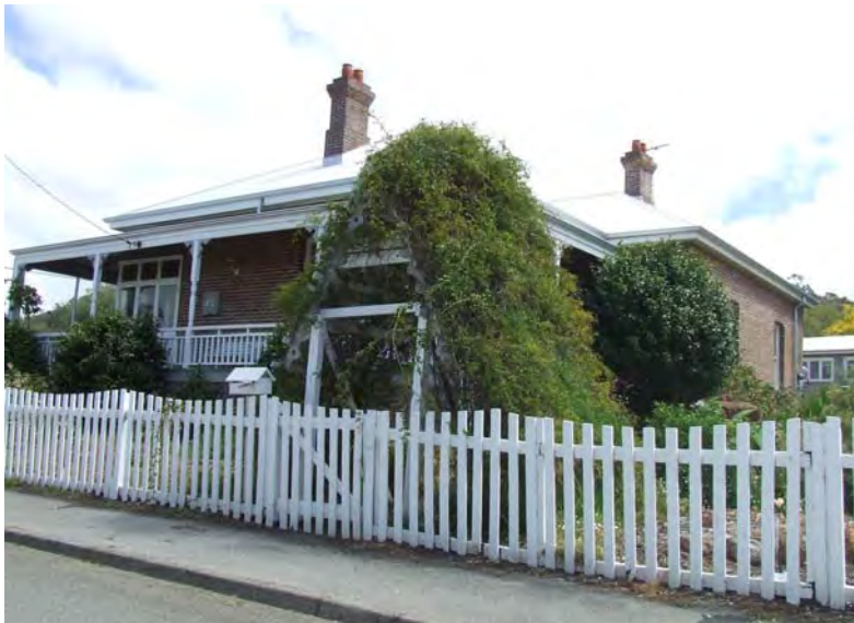
South-east elevation [H Munt 2018]
