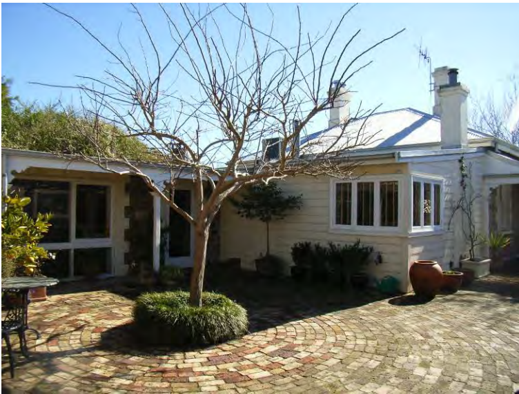
Rear addition [H Munt 2009]
