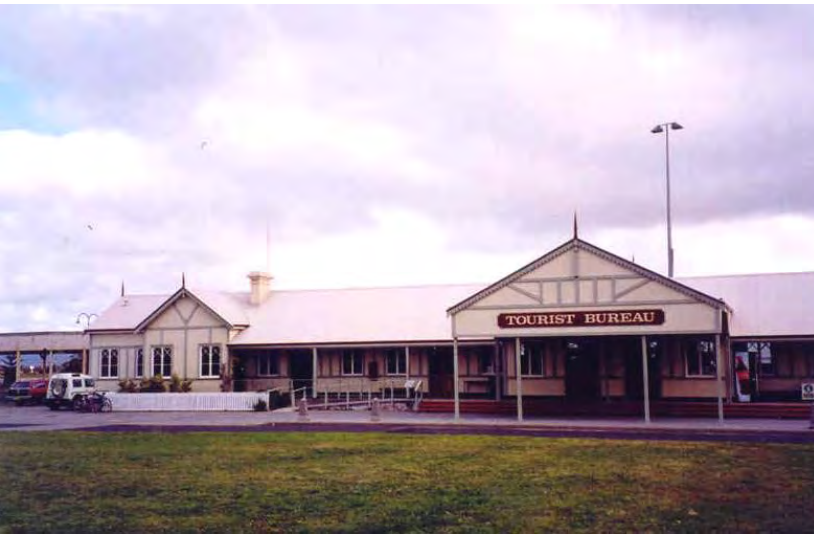
Railway Station north elevation [Heritage Today 2000]
