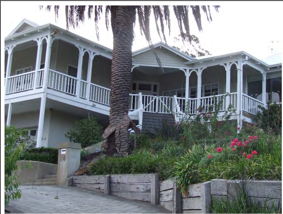
28-30 Cliff Street detail of front elevation (south) [H Munt 2016]
