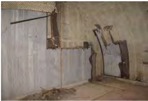
Engine Room [City of Albany, 2010]
