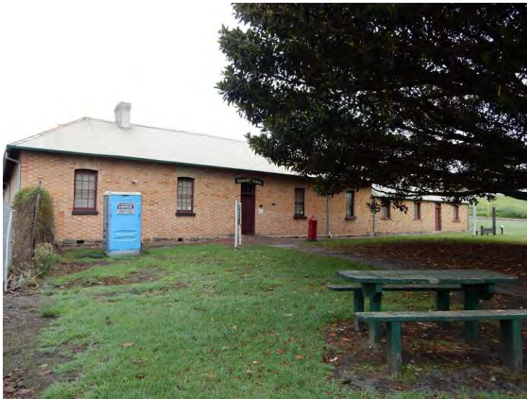
Front (east) elevation [H Munt 2017]
