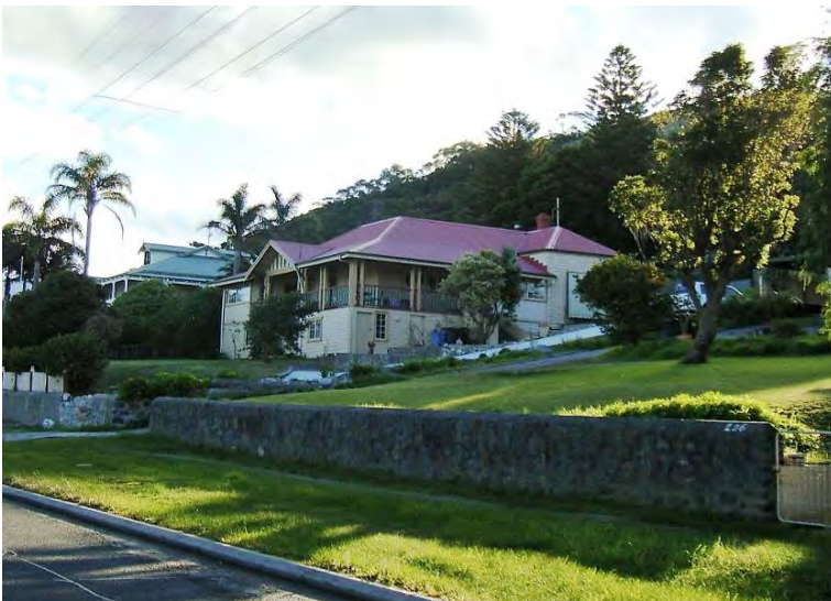
South-east elevation [H Munt 2008]
