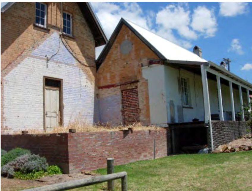
North east elevation during renovations 2009 [H Munt 2009]
