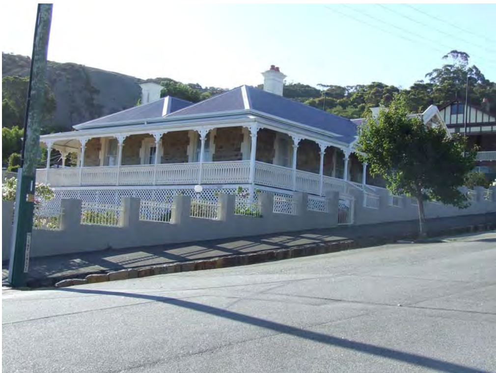
South-east elevation [H Munt 2018]
