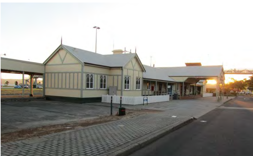
Railway Station north elevation [H Munt 2011]
