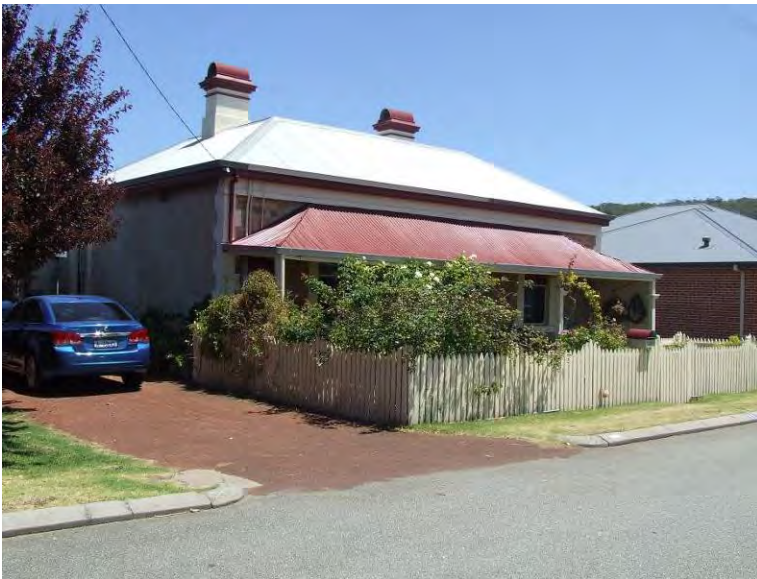
North-east elevation [H Munt 2017]
