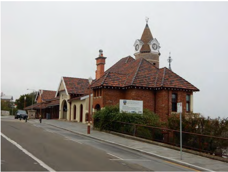
North west elevation from Stirling Tce [H Munt 2017]
