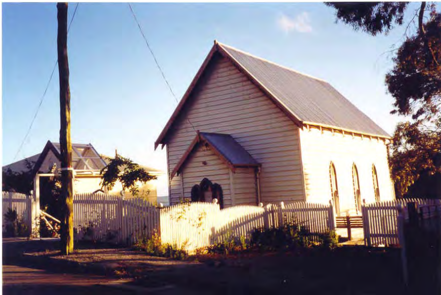
North-west elevation [Heritage Today 2000]
