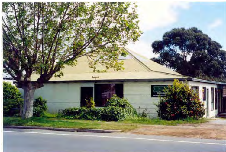
Prior to reconstruction works [Heritage Today 2000]
