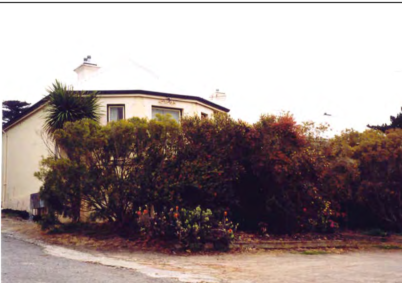
South-west elevation [Heritage Today 2000]
