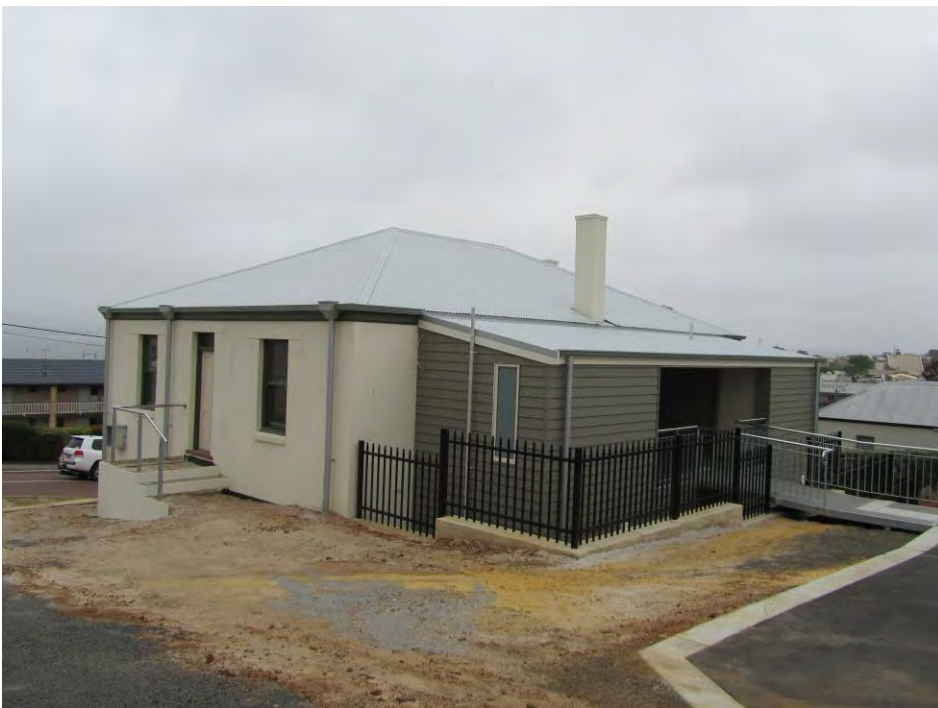
North-east façade [H Munt 2017]
