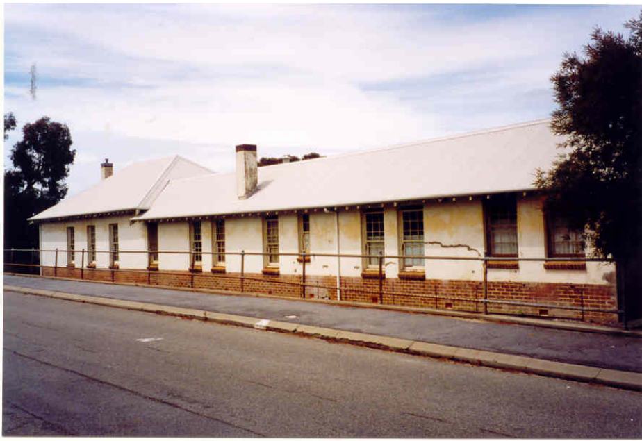
The later addition to the hospital on the east end now with metal roof and one chimney removed at the western end [Heritage Today 2000]
