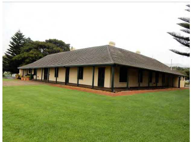
Residency - south-east elevation [H Munt 2017]
