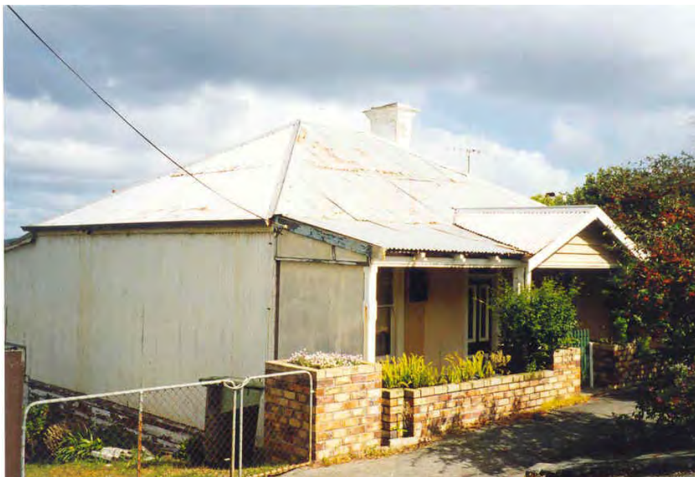
North-west elevation [Heritage Today 2000]
