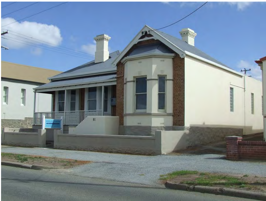
North-east elevation [H Munt 2016]
