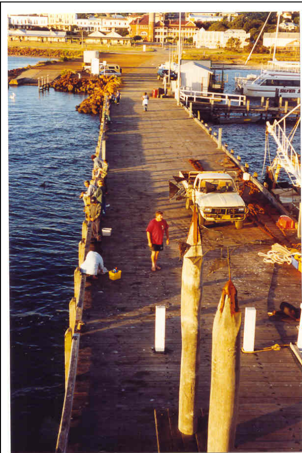
Albany Town Jetty – main section [ Heritage TODAY , 2000]
