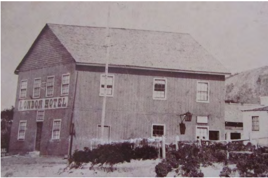
c1860 - the first two-storey timber London Hotel (fmr Hotel Chusan) [AHS]
