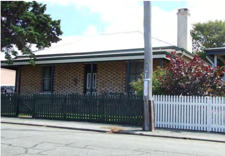
South-east elevation [H Munt 2018]
