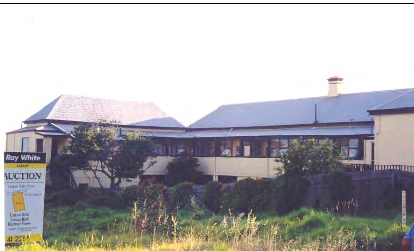
Showing the rear addition in 2000 [Heritage Today 2000]
