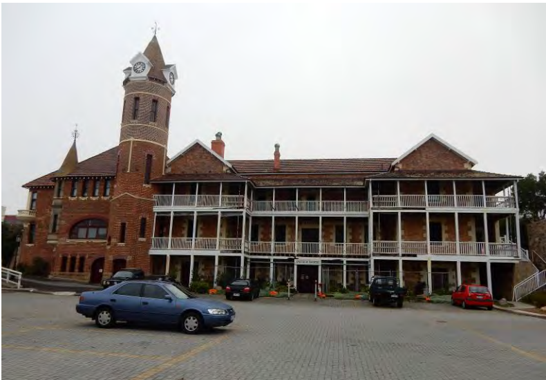
South elevation (rear)of the building [H Munt 2017]
