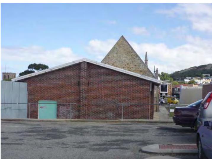
Rear elevation showing hall addition [H+H Architects, Scots Uniting Church Conservation Plan, 2010]
