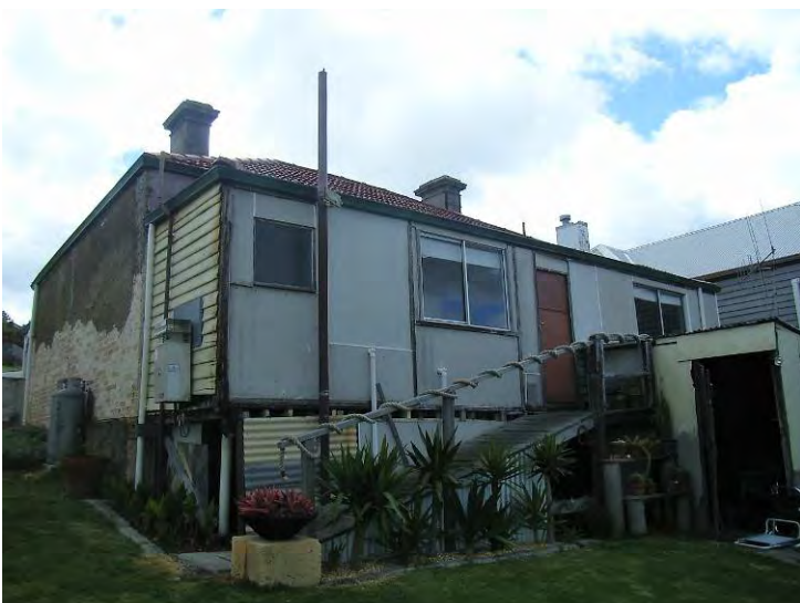
Before alterations and additions [H Munt 2007]
