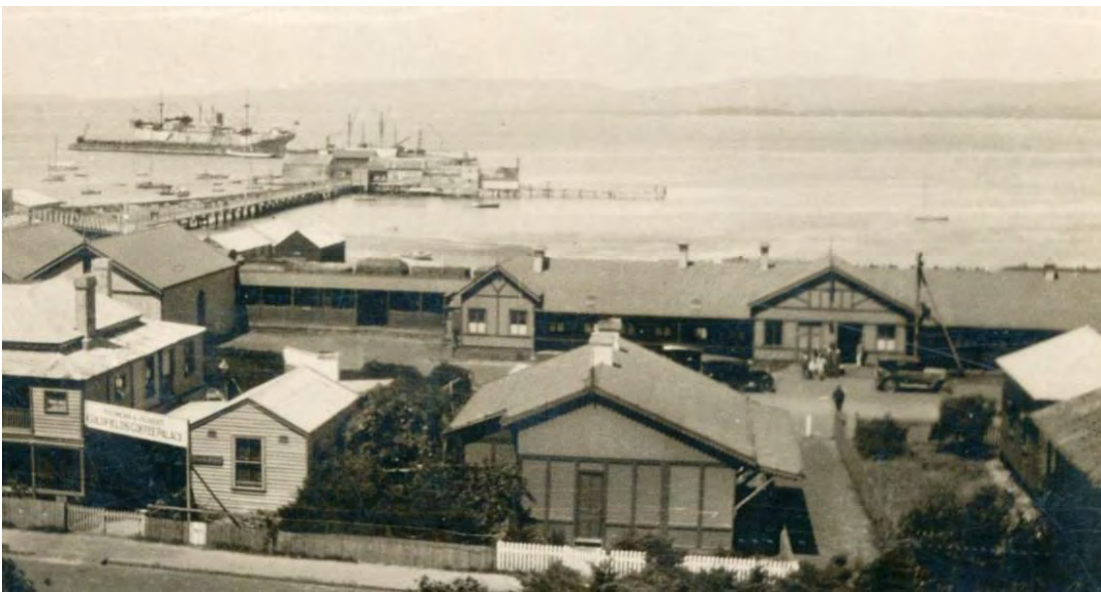
c1930s, Railway Station in background, north elevation [AHC P3966]
