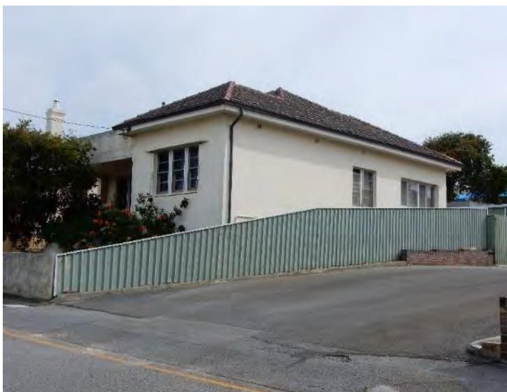
Officer's House south-east elevation [H Munt 2017]
