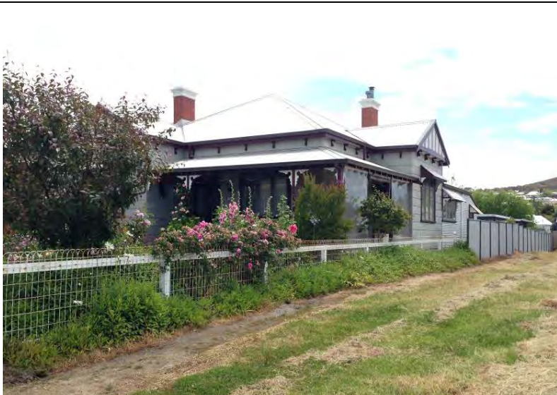
South-west elevation [H Munt 2016]
