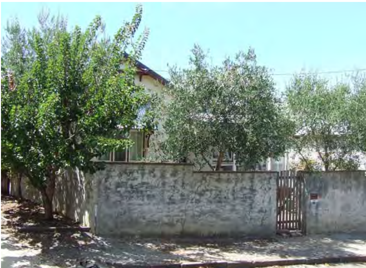
West elevation [H Munt 2018]
