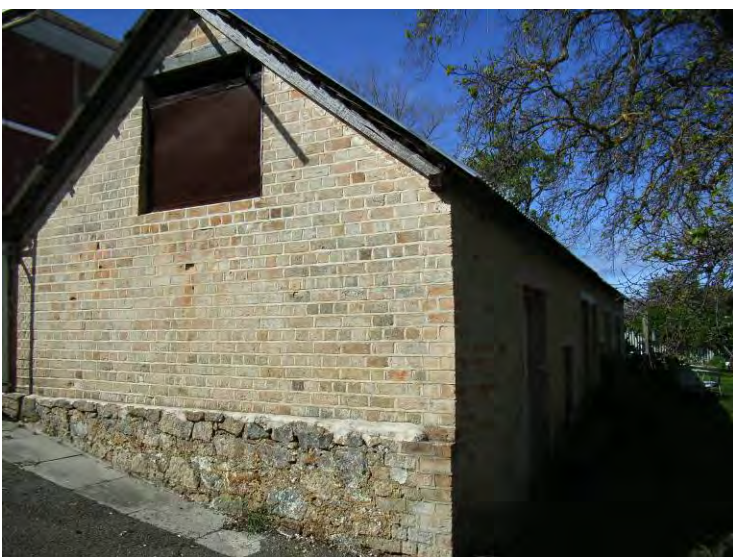
West elevation [H Munt 2008]
