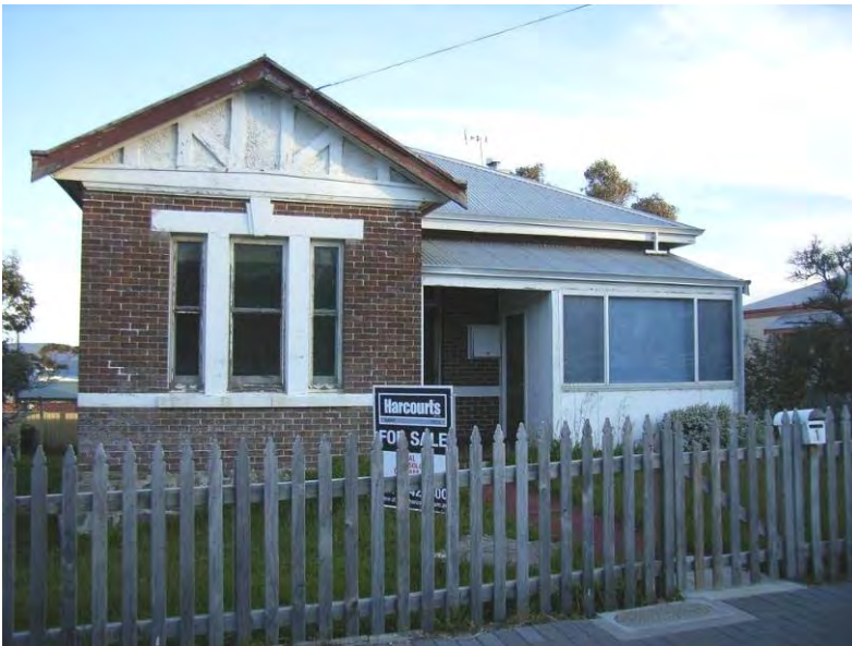
Sergeant's Quarters (fmr) – 1 Duke Street [H Munt 2010]
