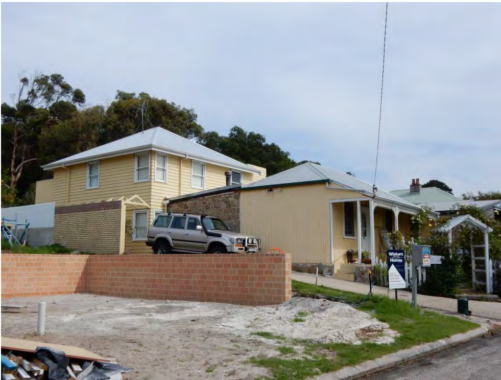
North-east elevation showing addition at rear [H Munt 2017]
