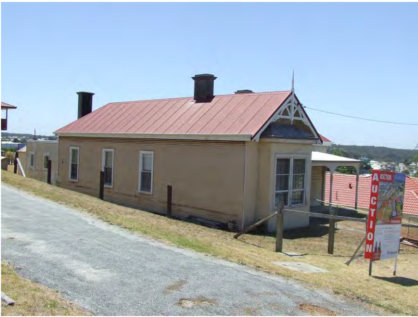
West elevation [H Munt 2017]
