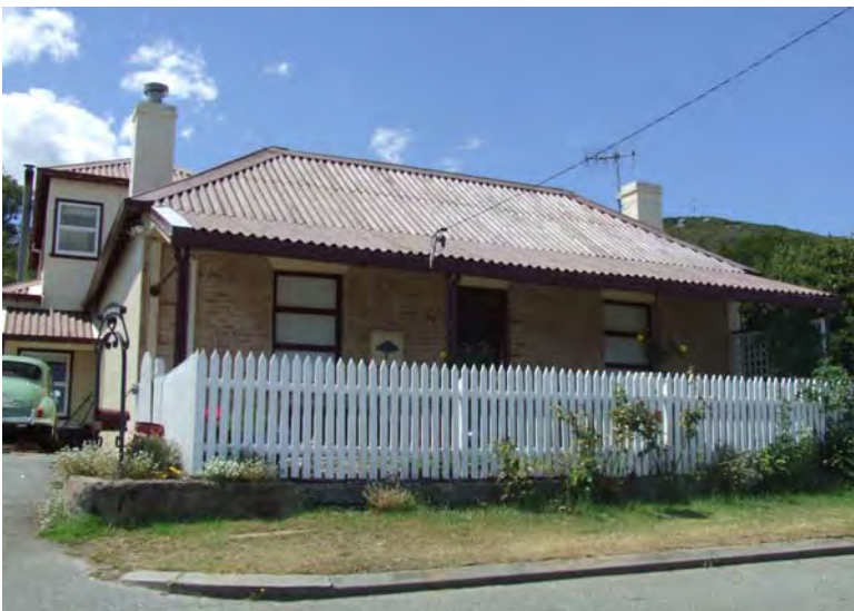
South-west elevation showing two storey rear addition [H Munt 2018]
