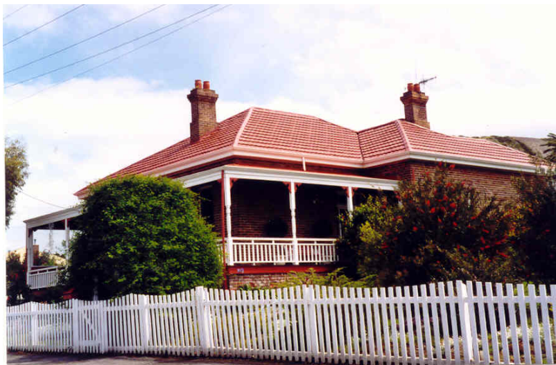
South-east elevation – note former tiled roof [Heritage Today 2000]
