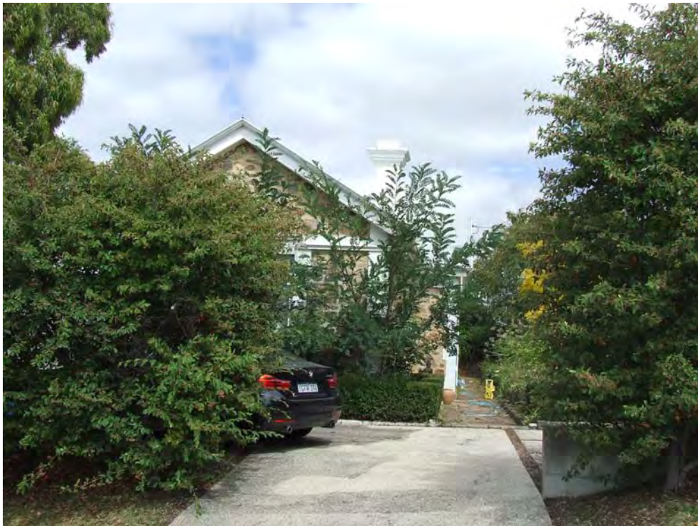
East elevation – note the house is now obscured by mature plantings [H Munt 2018]
