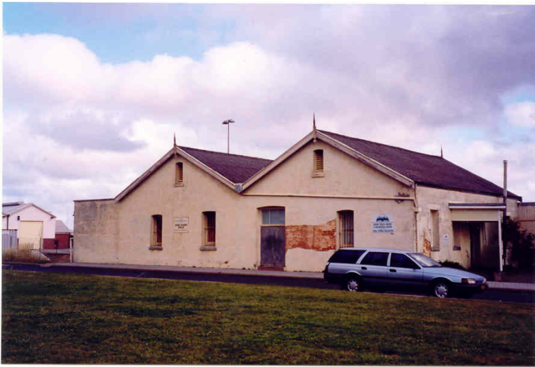
Railway Station Bond Store north elevation [Heritage Today 2000]
