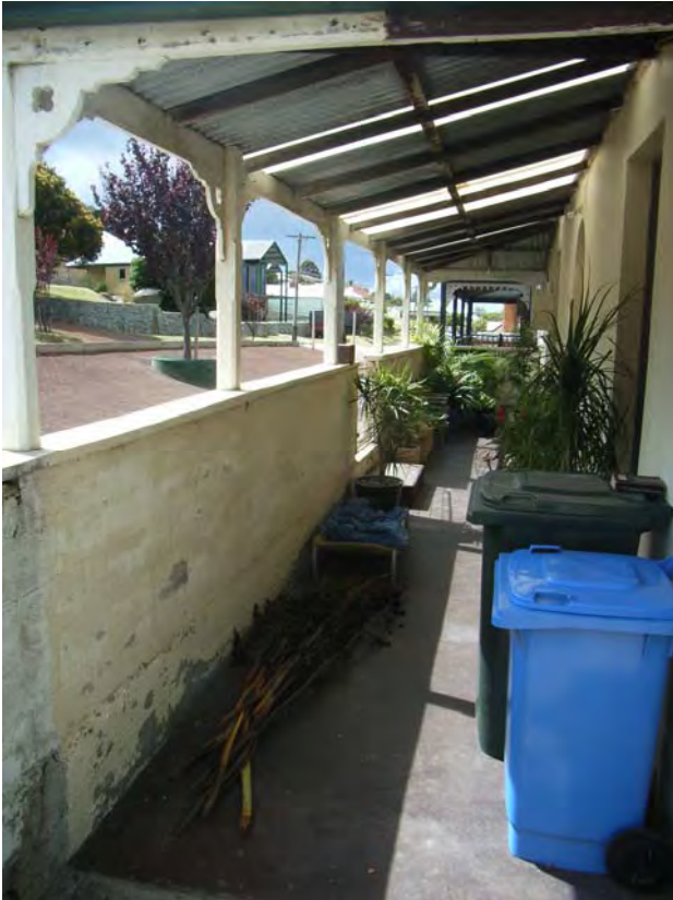
Before alterations and additions [H Munt 2007]
