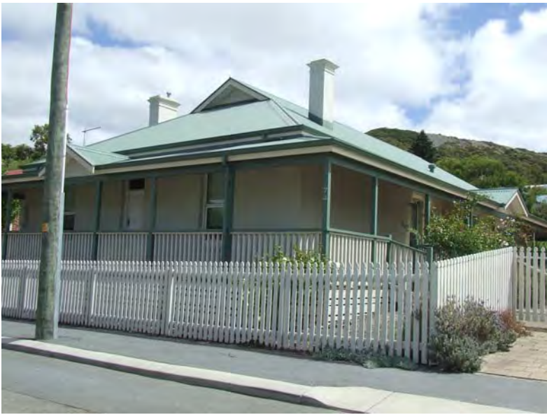
South-east elevation [H Munt 2018]
