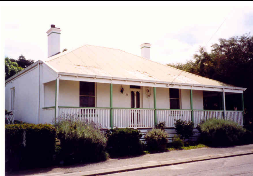
South-west elevation [Heritage Today 2000]
