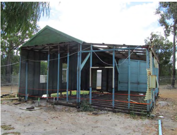
2012 demolition/reconstruction works [H Munt 2012]
