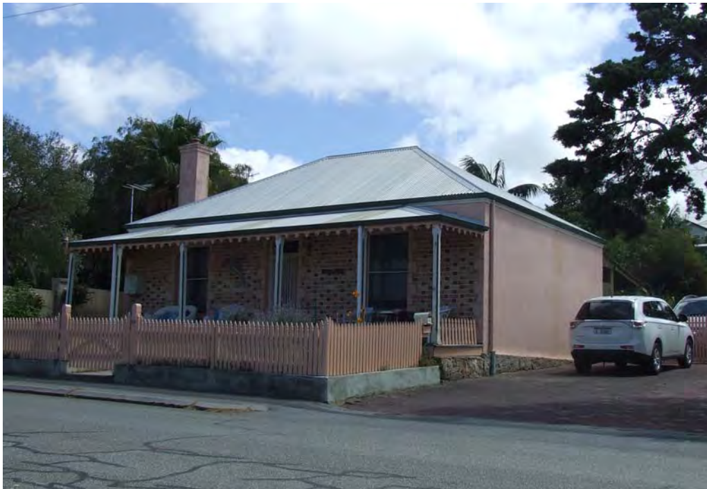
South-east elevation [H Munt 2018]
