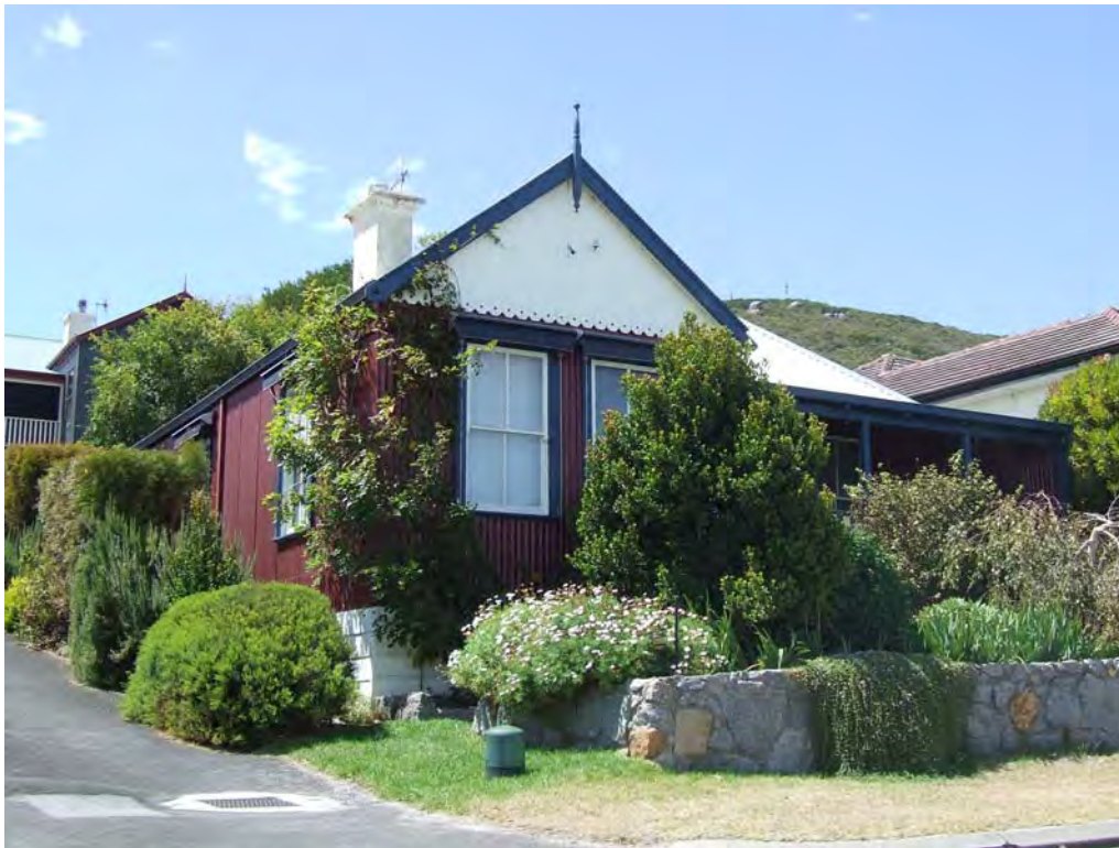
South-west elevation – note the change to external cladding, apron cladding and front window [H Munt 2018]
