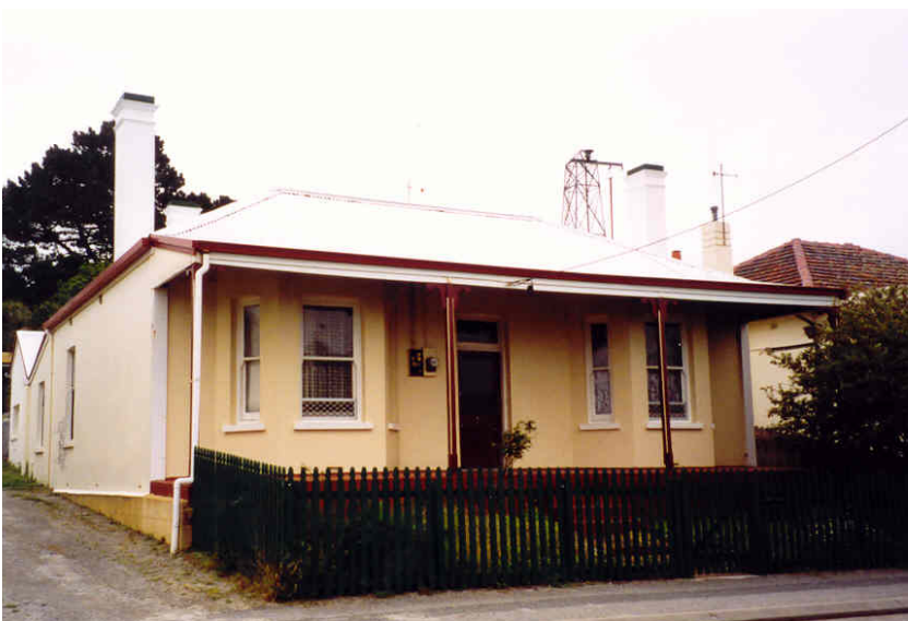
South-west elevation [Heritage Today 2000]
