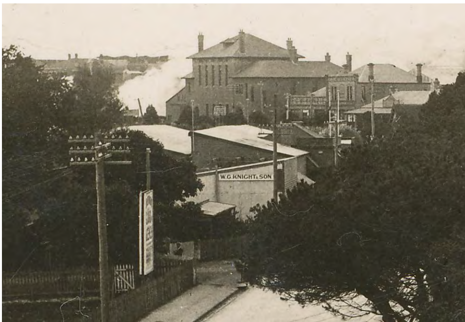
1920, looking west along Lower Stirling Tce, note the sawtooth roof [AHC P2073]
