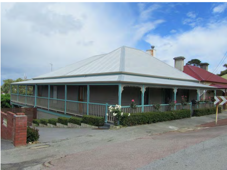
South-east elevation [H Munt 2010]
