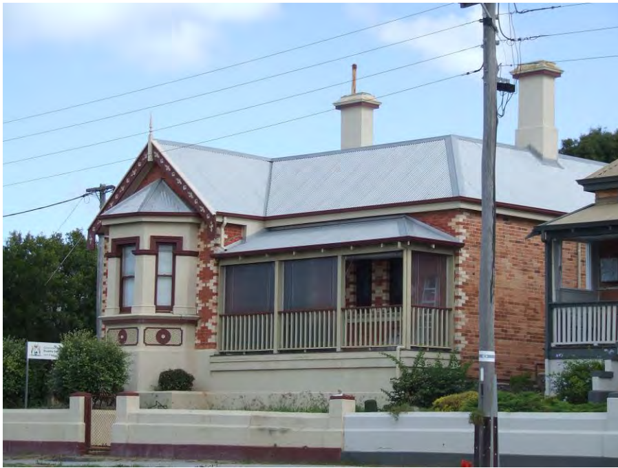
North-east elevation [H Munt 2016]
