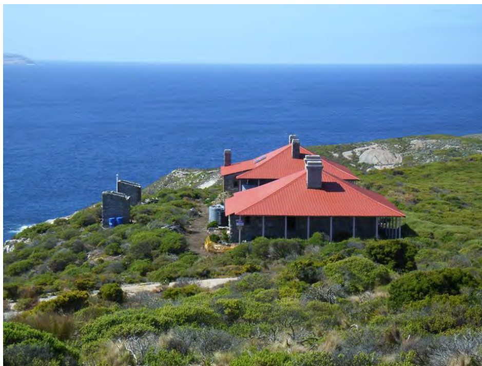
Lighthouse keepers' cottage 1902 & 1908 [H Munt 2008]
