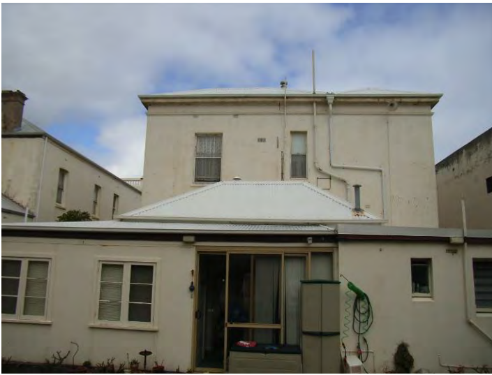
Rear elevation [H Munt 2008]
