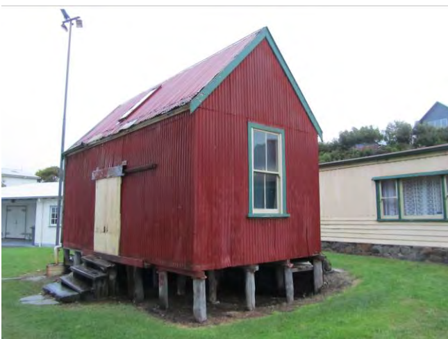
Net Shed – south-east elevation [H Munt 2011]
