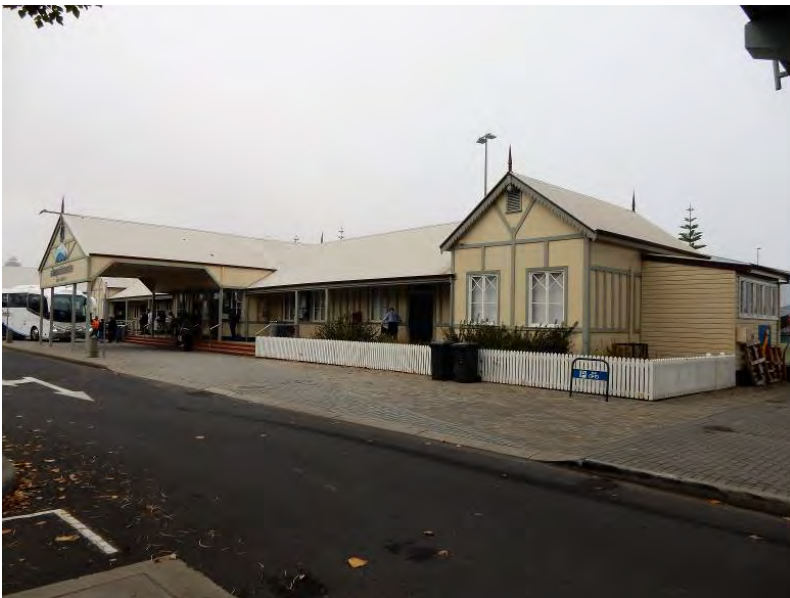
Railway Station north elevation [H Munt 2017]
