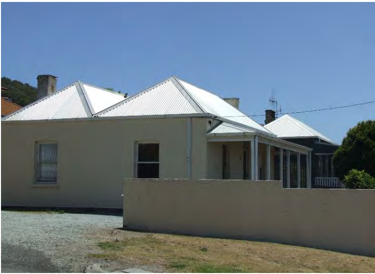
South-east elevation [H Munt 2016]
