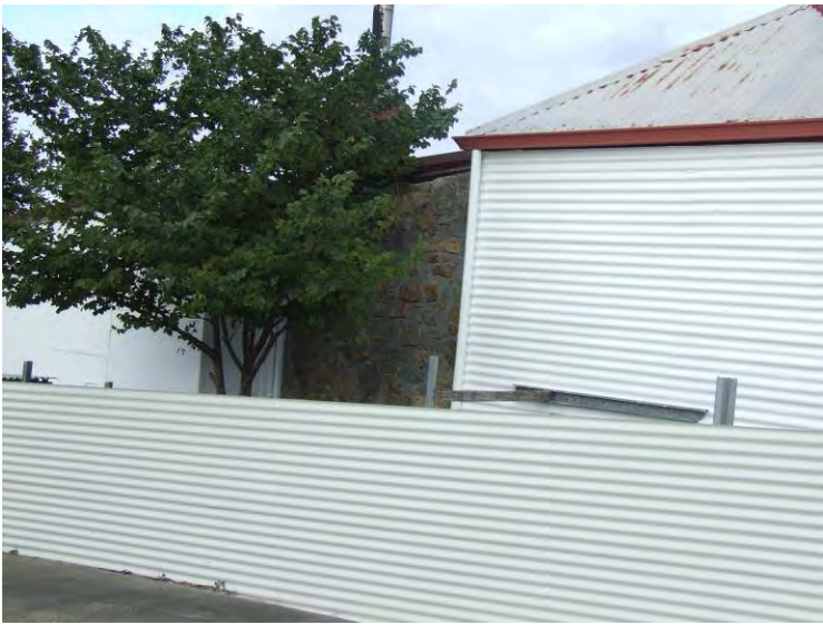
Detail of stone skillion lean-to [H Munt 2017]
