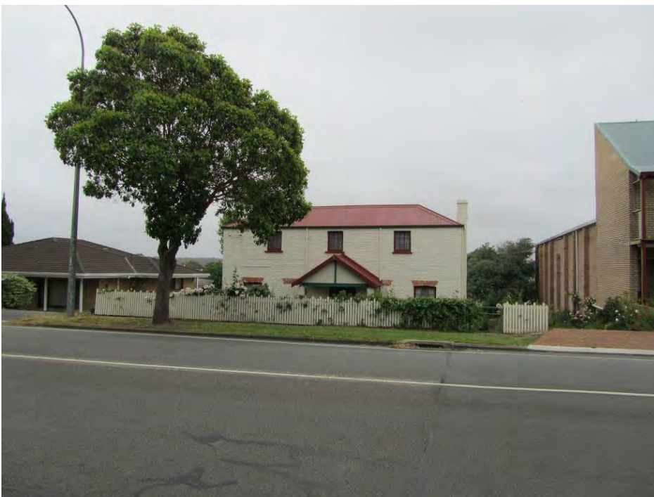
Front elevation from Middleton Rd [H Munt 2015]
