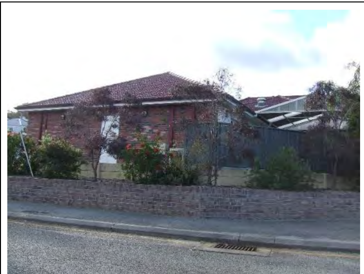
Fire Station, later additions at Vancouver Street elevation (south) [H Munt 2016]
