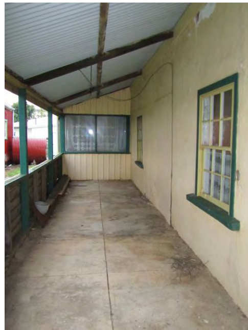
South verandah [H Munt 2011]
