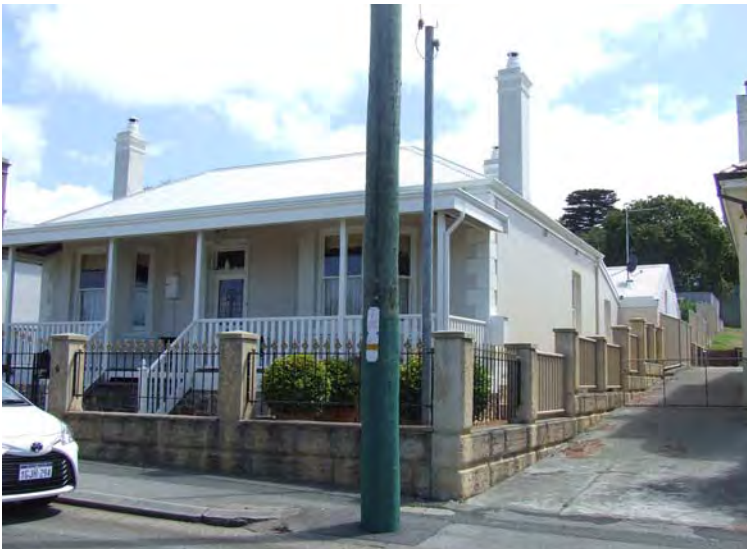
South-east elevation [H Munt 2018]
