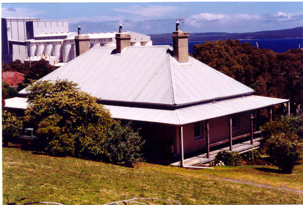
North-west elevation [Heritage Today 2000]
