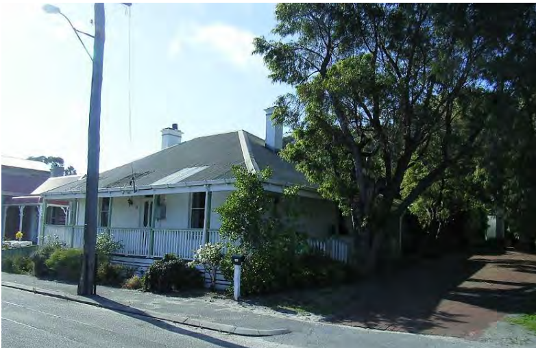
South-east elevation [H Munt 2008]
