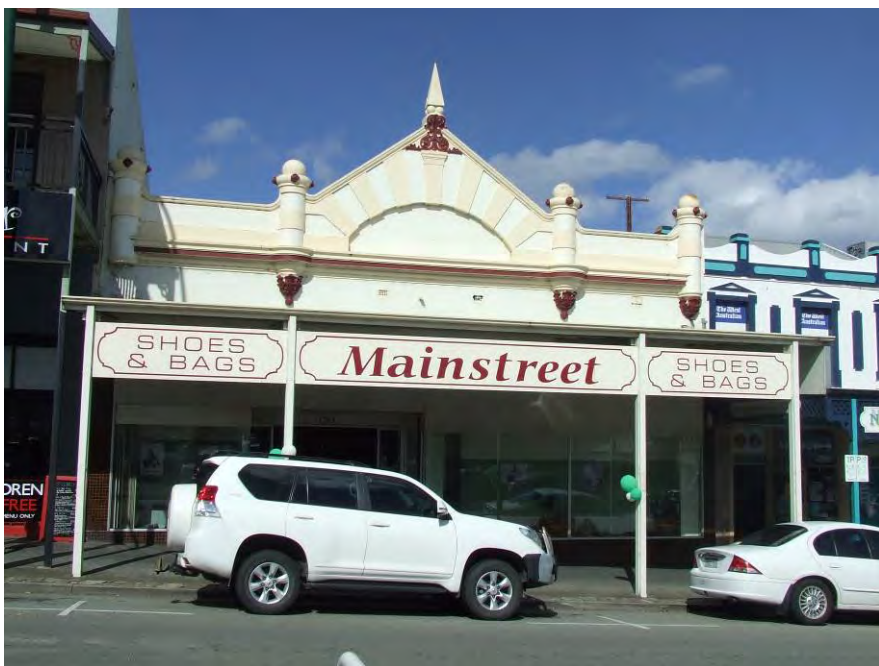
The single storey adjoining shop to the south of the original 2 storey St Albans Buildings [H Munt 2016]
