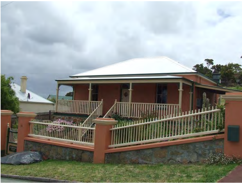
South-east elevation [H Munt 2015]
