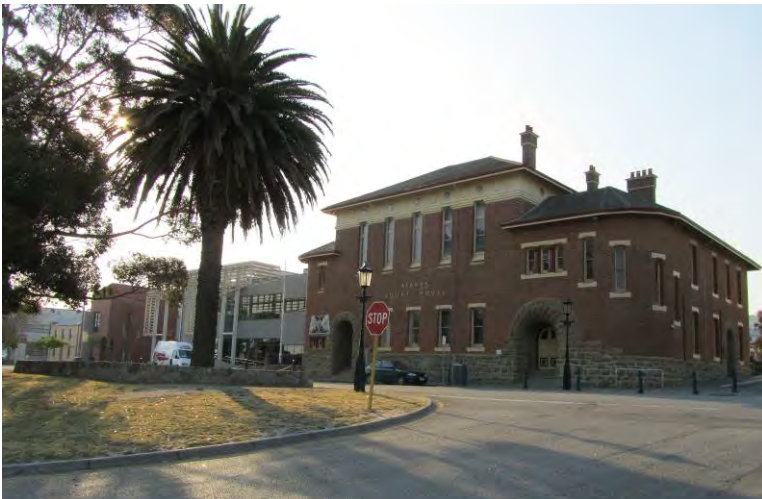
Court House showing south-east elevation [H Munt 2010]
