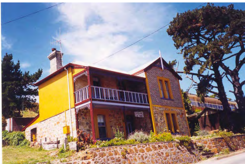
South-west elevation – showing former colour scheme and pine trees [Heritage Today 2000]
