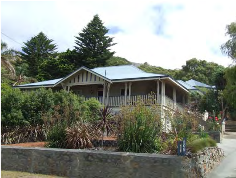
South-east elevation [H Munt 2018]
