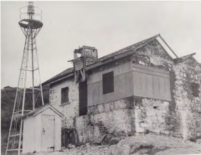
Point King Lighthouse [Albany History Collection 029661]
