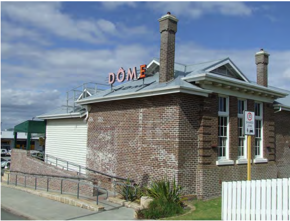
As Dome Café - north elevation [H Munt 2016]
