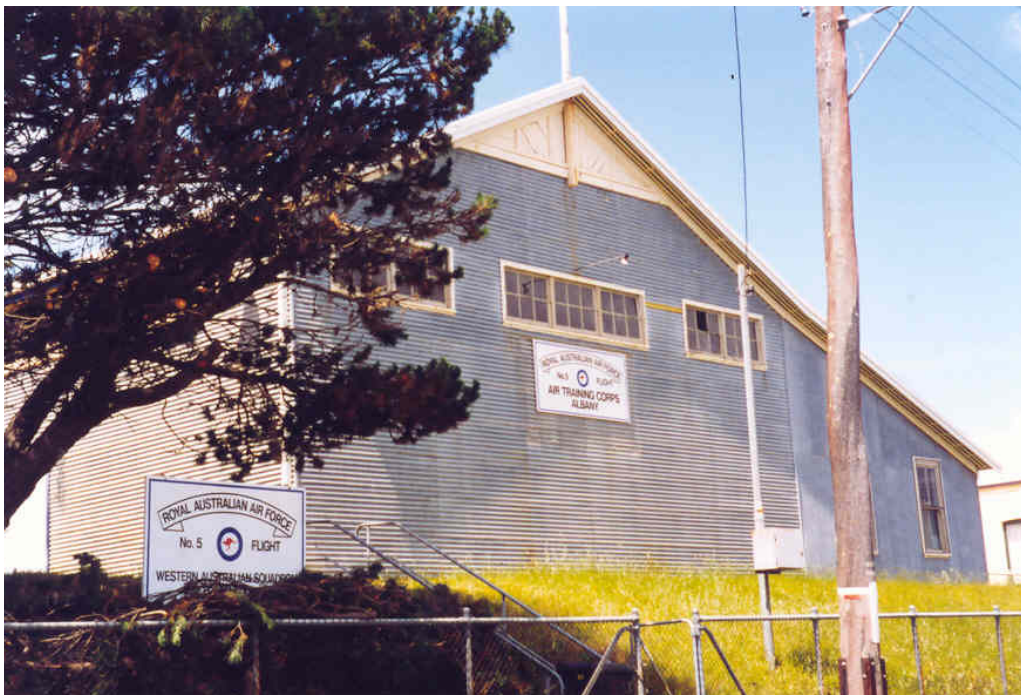
North-west elevation from Spencer Street [Heritage Today 2000]
