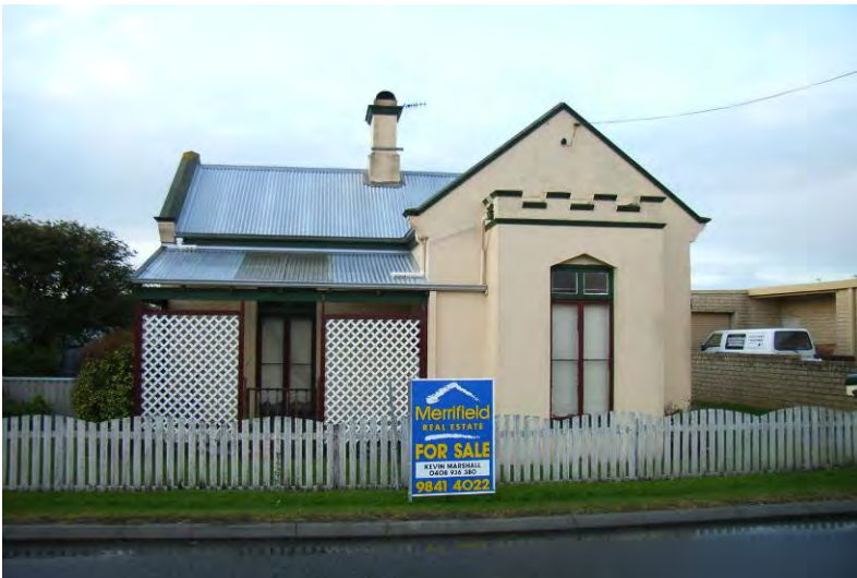
Showing former colour scheme [H Munt 2007]
