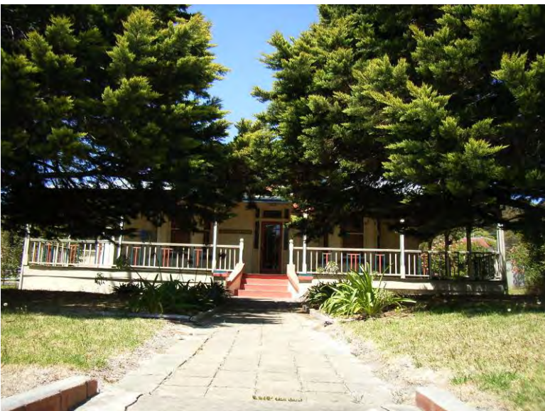
St Joseph's Lodge New Camfield (Parish Centre) [H Munt 2007]
