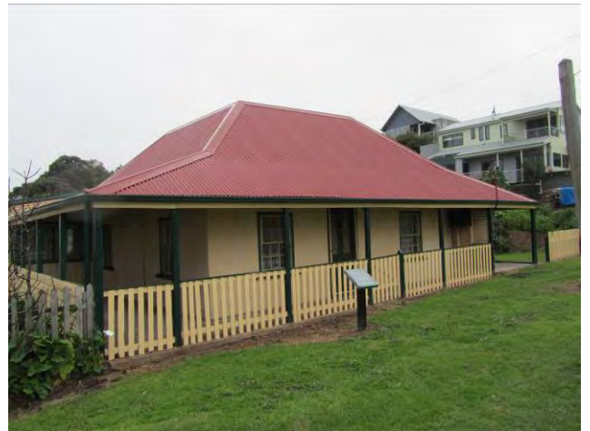
South-east elevation [H Munt 2011]
