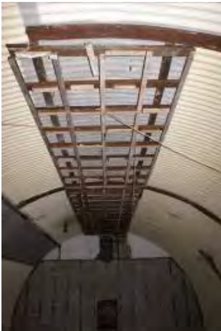
Ceiling detail in engine room [City of Albany, 2010]
