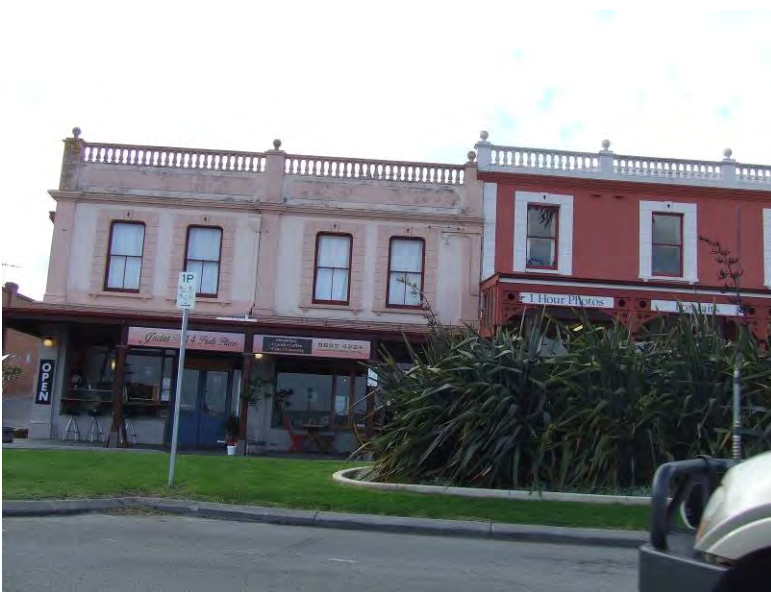
South elevation – western end [H Munt 2017]
