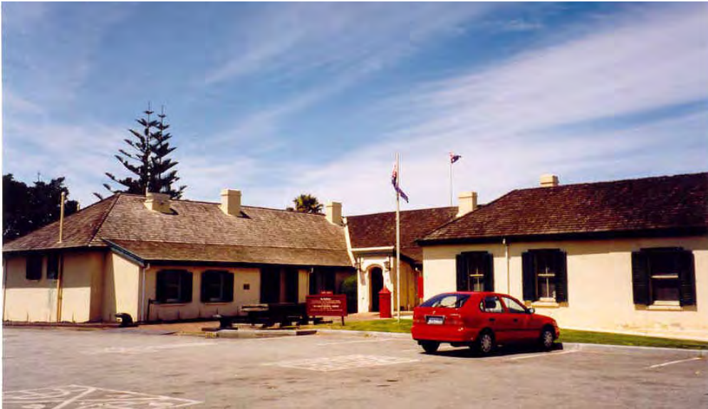
Residency north/north-west elevation [Heritage Today 2000]
