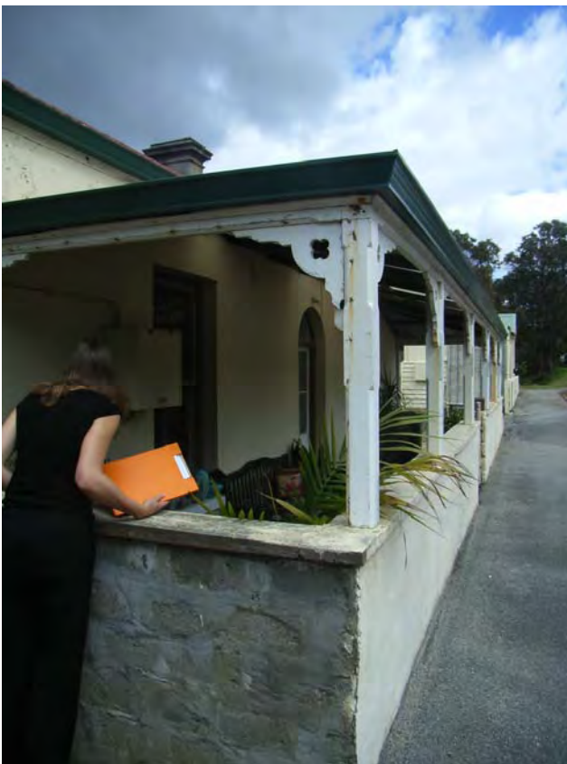
Before alterations and additions [H Munt 2007]
