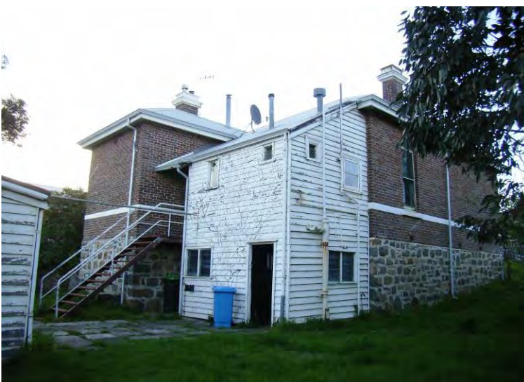
Sergeant's Quarters (fmr), 1 Duke Street, rear elevation [H Munt 2010]
