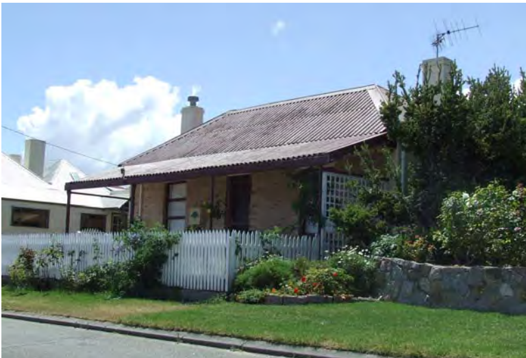
South-east elevation [H Munt 2018]
