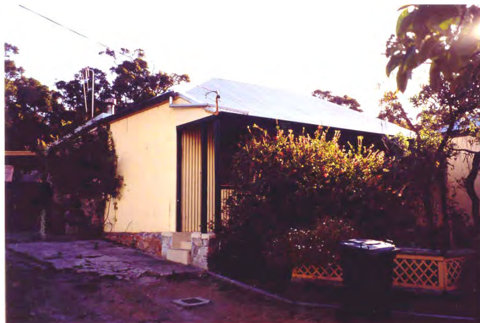
North-east elevation before addition [Heritage Today 2000]
