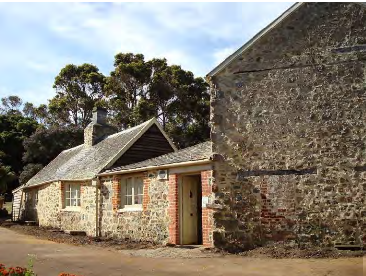
2009, main stone house (right) and kitchen (left) [H Munt 2009]
