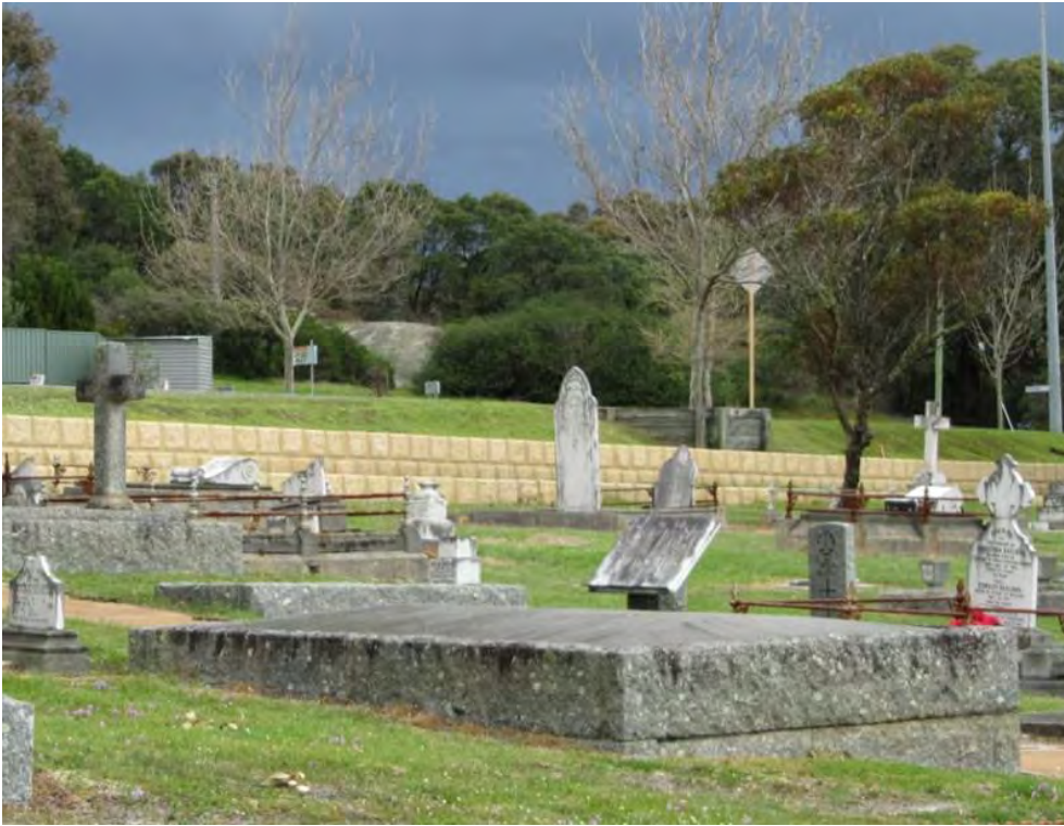
Northern section showing newly installed limestone retaining wall [H Munt 2012]
