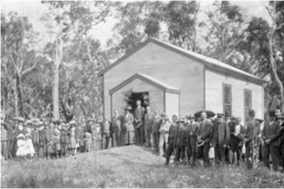
21 December 1912, official opening of Kalgan Hall, note raised earthen ramp in front of porch entrance, and details of windows and vents at west side wall. [photograph included in Conservation Plan, courtesy Chris Andrews, and Kalgan Settlers' Association]
