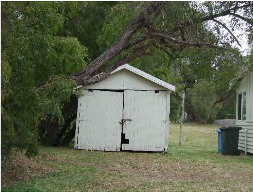
Garage - west of house [H Munt 2015]
