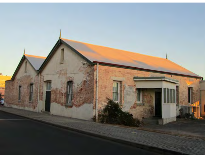
Bond store prior to conservation works [H Munt 2011]
