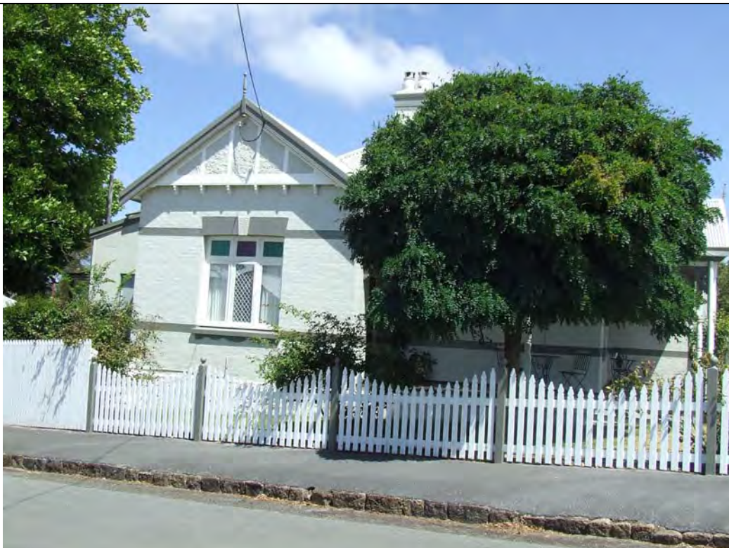
West elevation (from Cuthbert St) [H Munt 2018]
