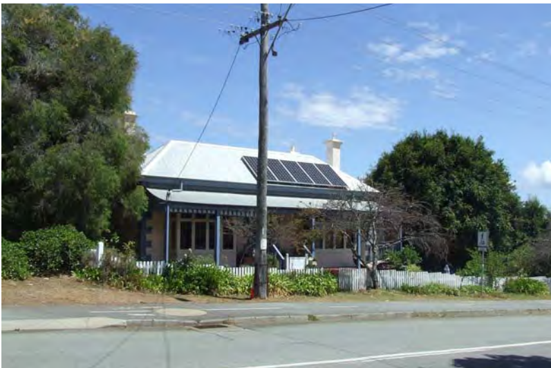
North-east elevation [H Munt, 2018]
