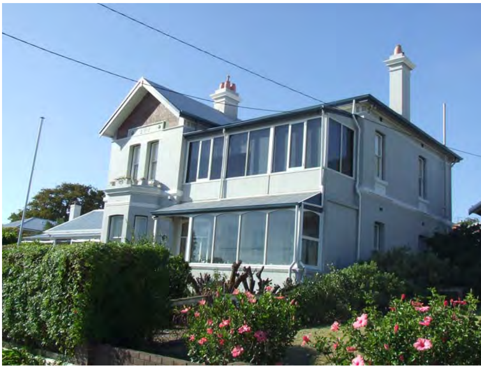
South-east elevation showing rendered wall on east [H Munt 2018]
