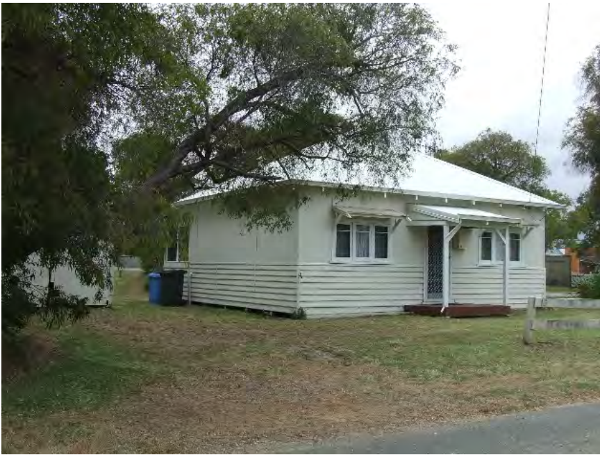
Front elevation south-west [H Munt 2015]
