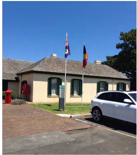
Residency - north elevation [H Munt 2017]
