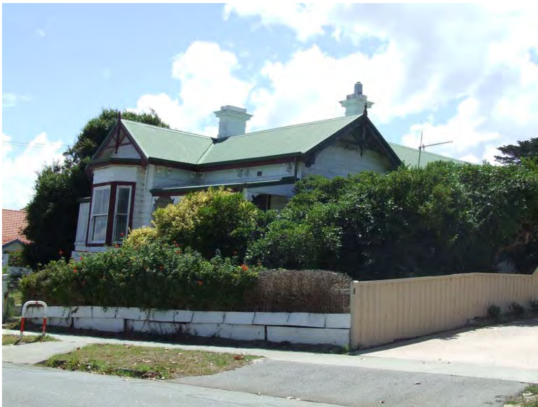
South-east elevation [H Munt 2018]
