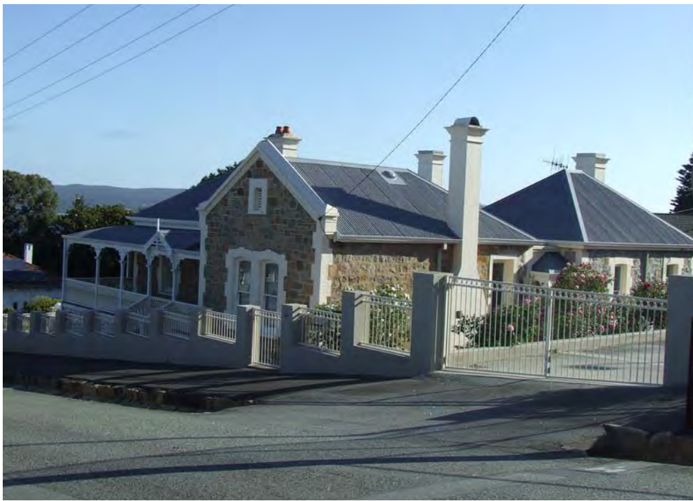
North-east elevation [H Munt 2018]
