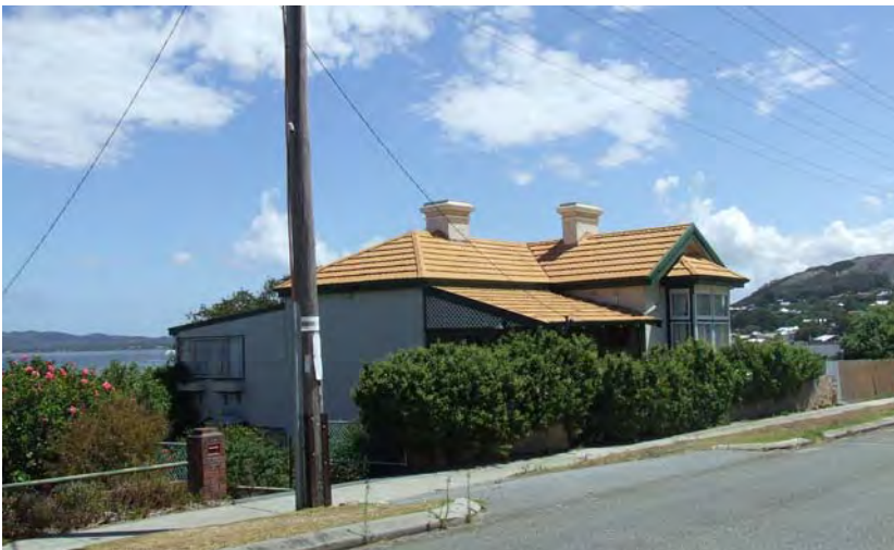
North-east elevation [H Munt 2018]
