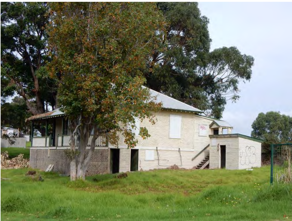
North elevation [H Munt 2017]
