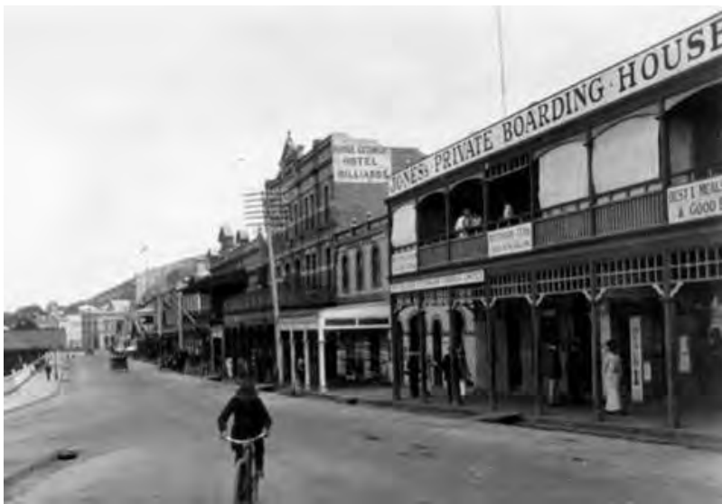
1915 showing double storey timber verandah [SLWA 0531D]
