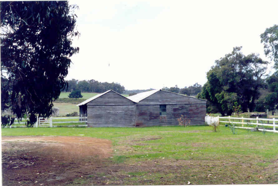
Outbuilding [Heritage Today 2000]
