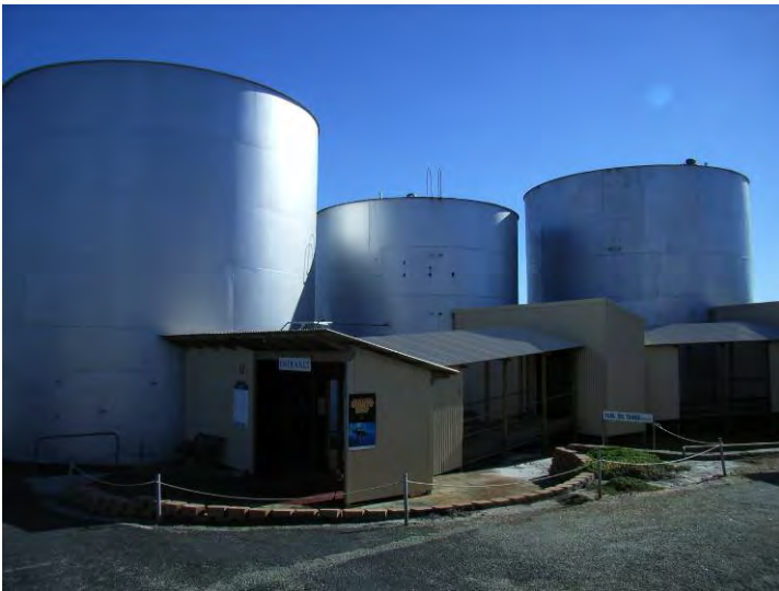
Tanks converted into multi-media exhibition spaces [H Munt 2007]
