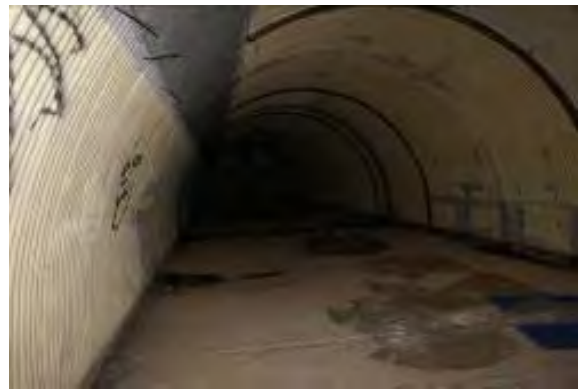
Tunnel/bunker [City of Albany, 2010]
