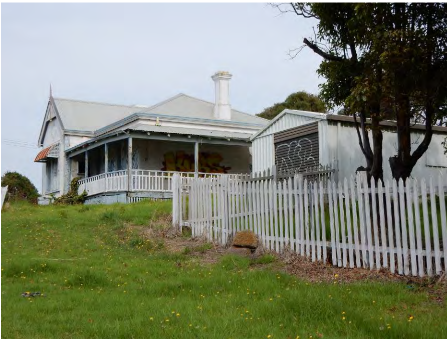
North elevation [H Munt 2017]
