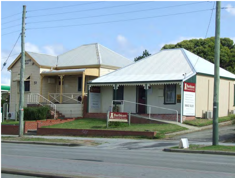
North-east elevation [H Munt 2017]
