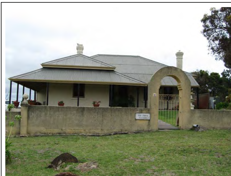
Caretaker's House [H Munt 2011]
