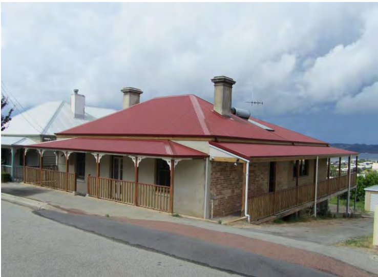
After alteration and additions – note new roof, timber balustrading to front verandah and rear addition with side verandah [H Munt 2010]
