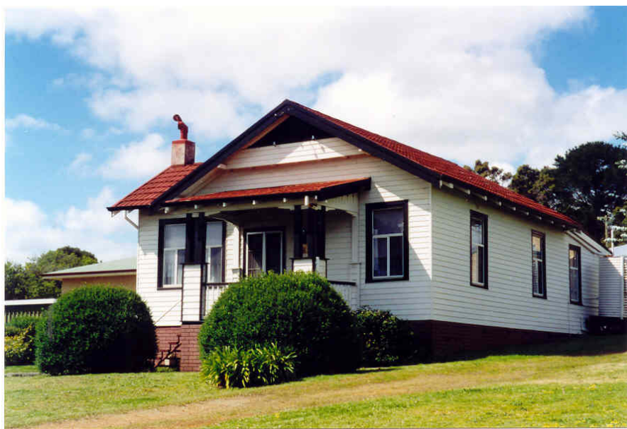
North-west elevation [Heritage Today 2000]
