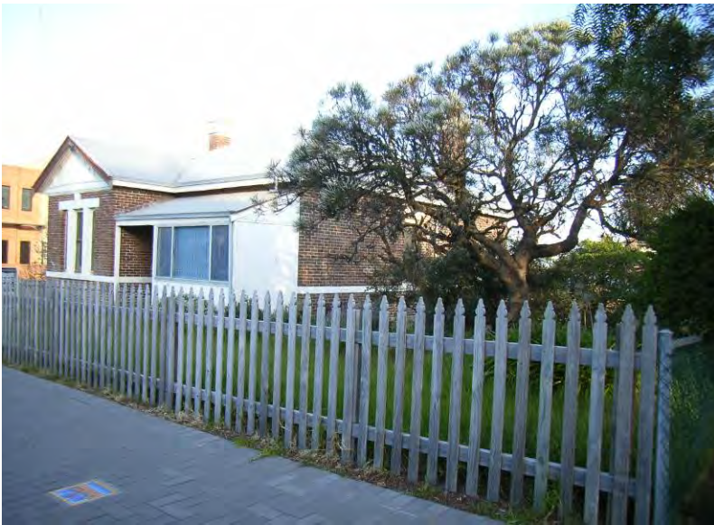
Sergeant's Quarters (fmr), 1 Duke Street, [H Munt 2010]
