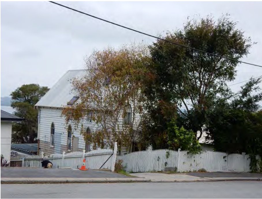
North-east elevation [H Munt 2017]
