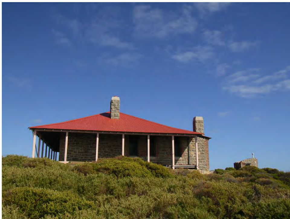
Lighthouse keepers' cottage [H Munt 2008]
