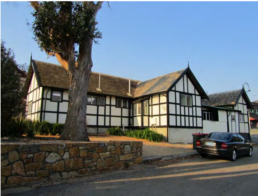
Rear (south) elevation [H Munt 2010]
