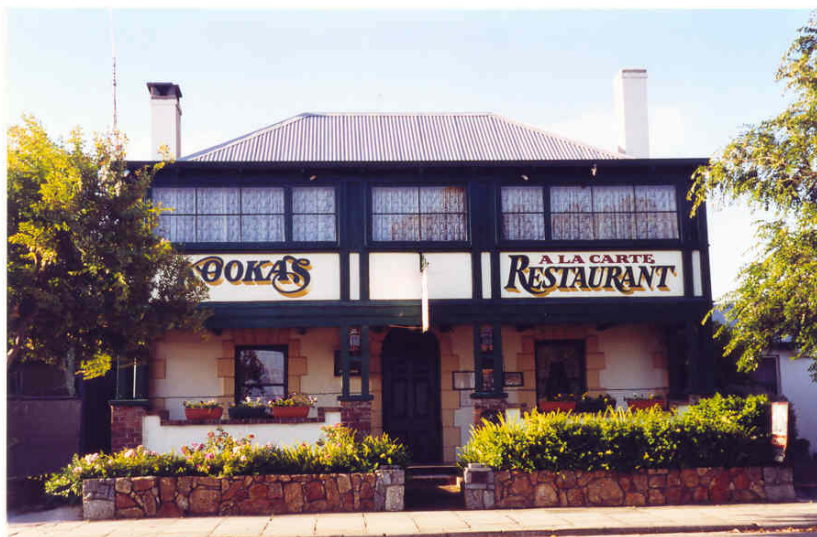
Kookas, prior to conservation works [Heritage Today 2000]
