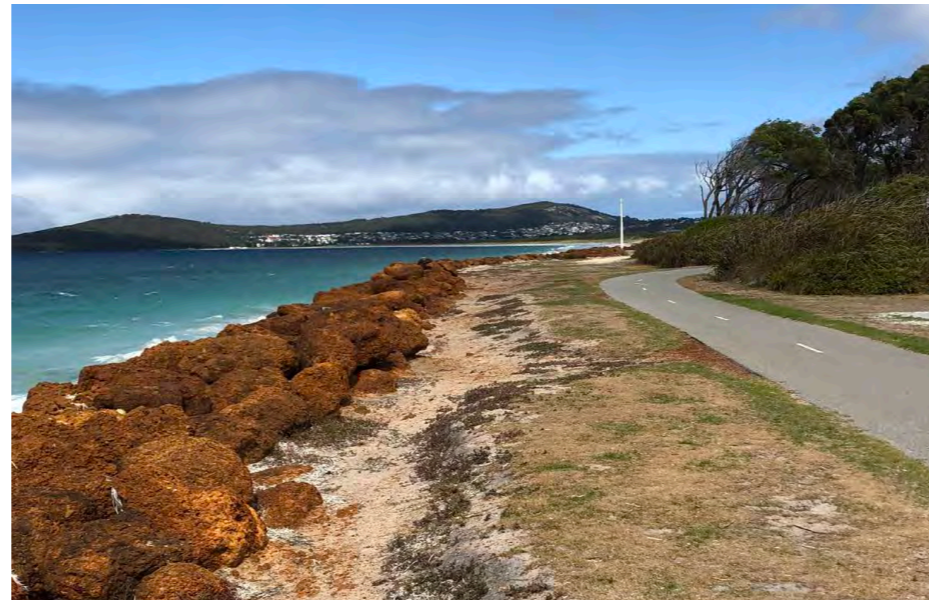
1. Existing coastal structure
