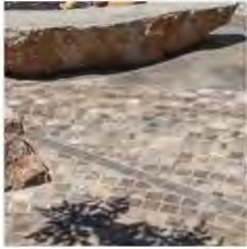
Radial paving patterns using local granite stone
