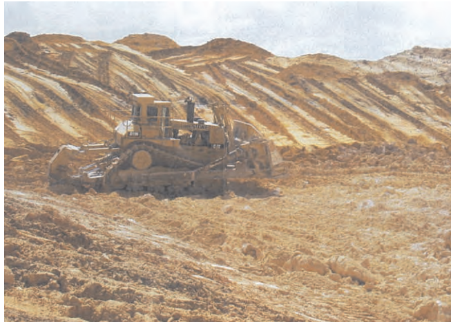
Bulldozer ripping and crushing limestone
