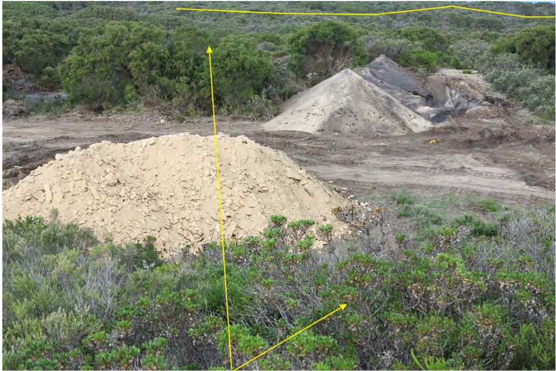
Rehabilitation at the old limestone pit
