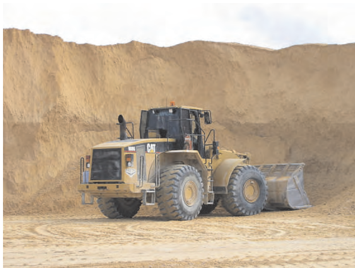
Loader, loading limestone
