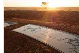
'DIRECTIVE SIGNAGE' IN NEW PATH WAY CAST IN LIME STONE COLOURED CONCRETE TO FORM DISTINGUISHED SECTION IN NEW LIME STONE WALK TRAIL (INDICATIVE LAYOUT)
