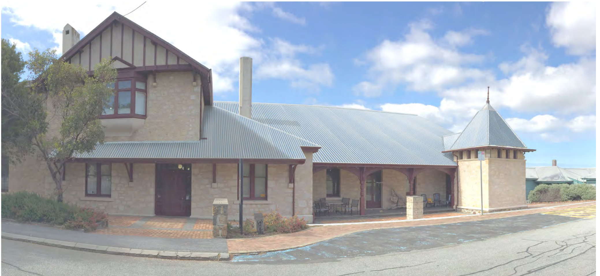
VANCOUVER ARTS CENTRE - GALVANISED CORRUGATED SHEETING ROOF OPTION
