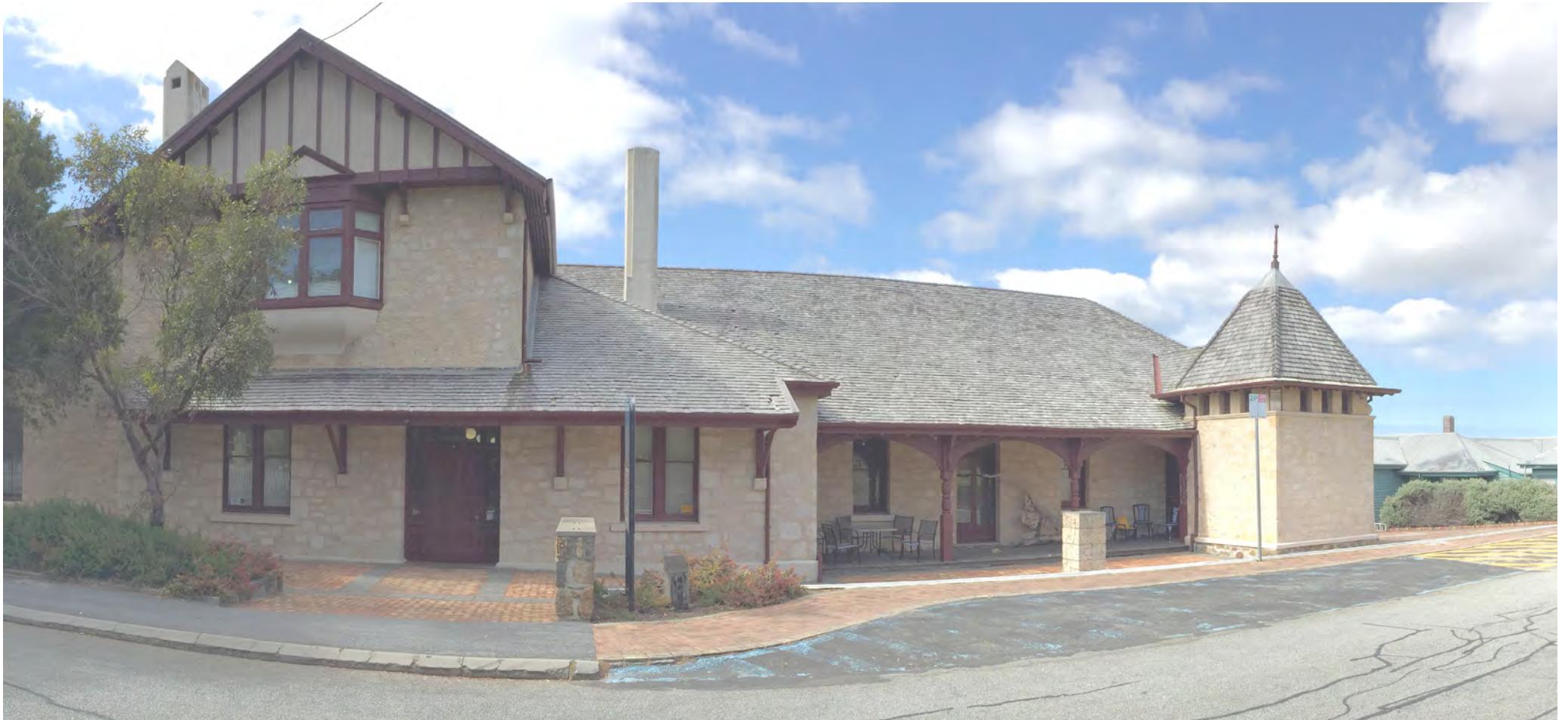
VANCOUVER ARTS CENTRE - EXISTING CONDITION
