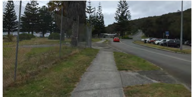
Figure 9: Existing Footpath Adjacent to MBAC along Adelaide Crescent
