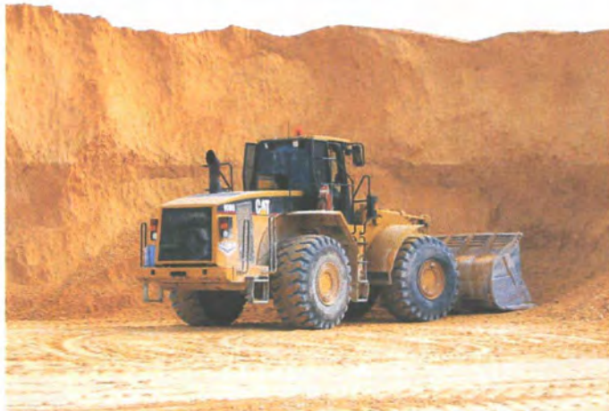
Loader, loading limestone
