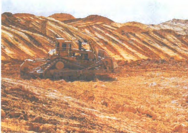
Bulldozer ripping and crushing limestone
