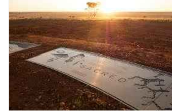
'DIRECTIVE SIGNAGE' IN NEW PATH WAY CAST IN LIME STONE COLOURED CONCRETE TO FORM DISTINGUISHED SECTION IN NEW LIMESTONE WALK TRAIL (INDICATIVE LAYOUT)
