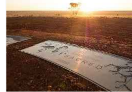
'DIRECTIVE SIGNAGE' IN NEW PATH WAY CAST IN LIME STONE COLOURED CONCRETE TO FORM DISTINGUISHED SECTION IN NEW LIME STONE WALK TRAIL (INDICATIVE LAYOUT)
