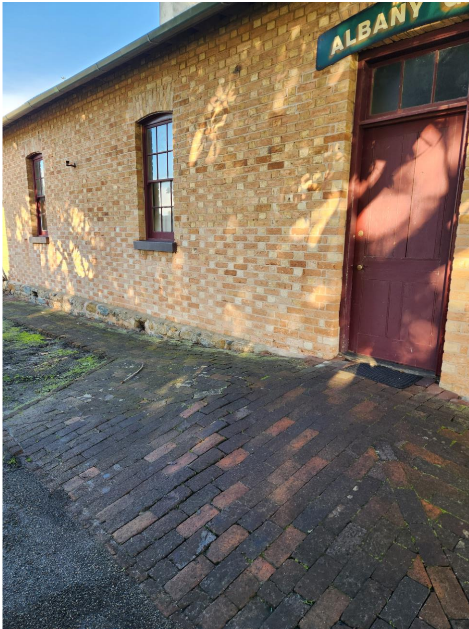
Fig.2 - View of the stem of the font (main) pedestrian entrance to the Old Goal building in Albany showing brick paving displaced by root development (photo taken 10/7/2024).
