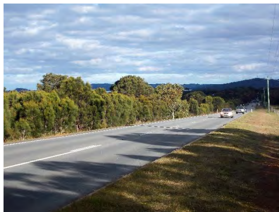
View of Lower King Road showing that a future intersection will have appropriate sight distances.
