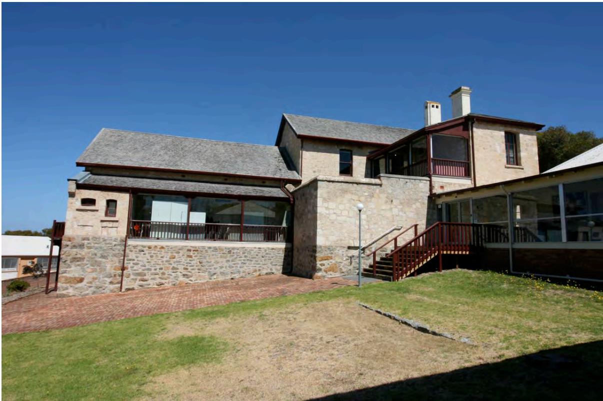
Photo 7 Vancouver Arts Centre – Albany Cottage Hospital (fmr): east façade
