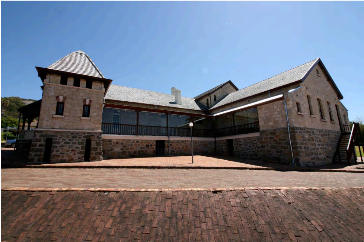
Photo 6 Vancouver Arts Centre – Albany Cottage Hospital (fmr): south (rear) façade
