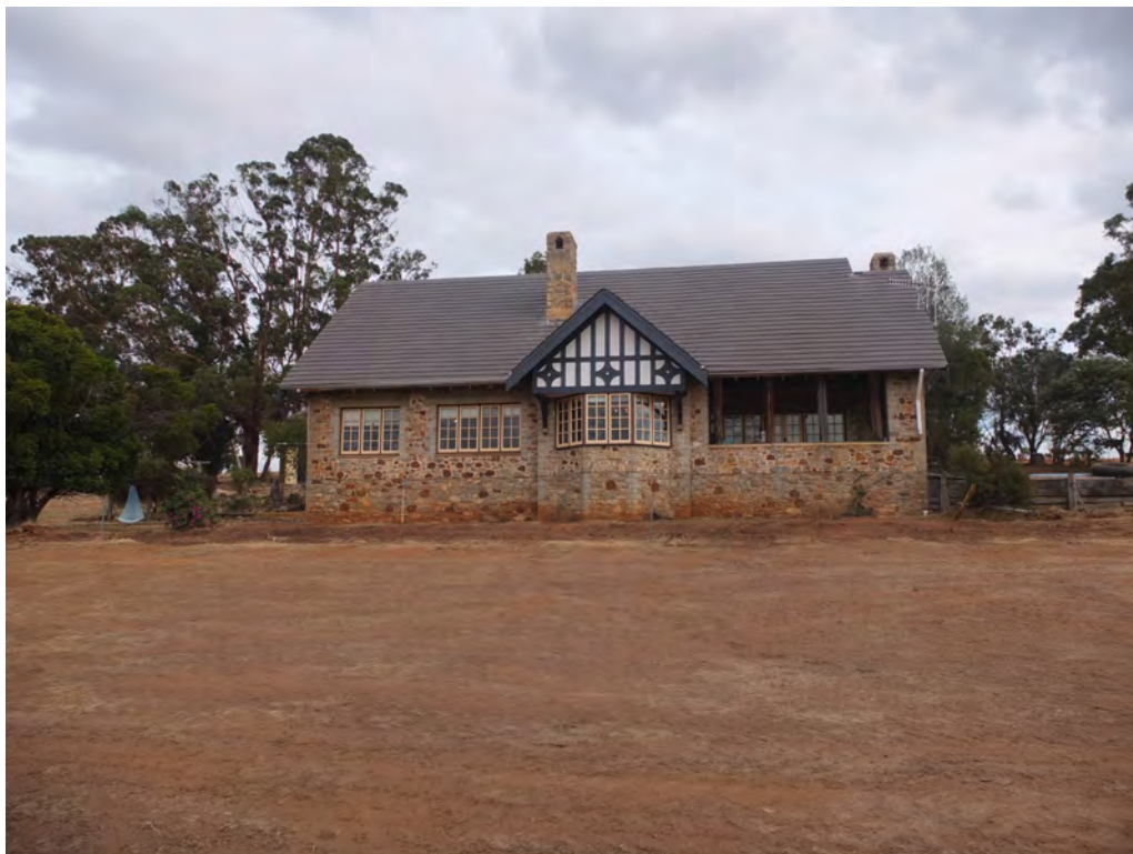
Photo 11 The same roof clad with Midland Brick Shingle Asphalt cover
