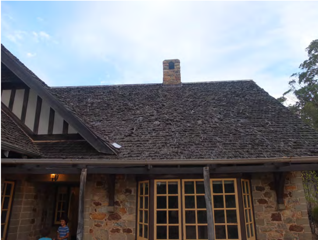
Photo 10 Midland Brick photo of house with shingle roof in very poor condition
