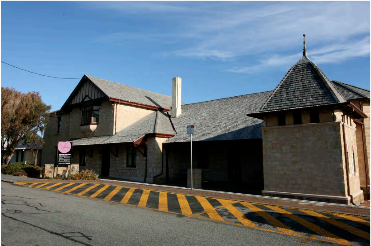
Photo 4 Vancouver Arts Centre – Albany Cottage Hospital (fmr): north (front) façade
