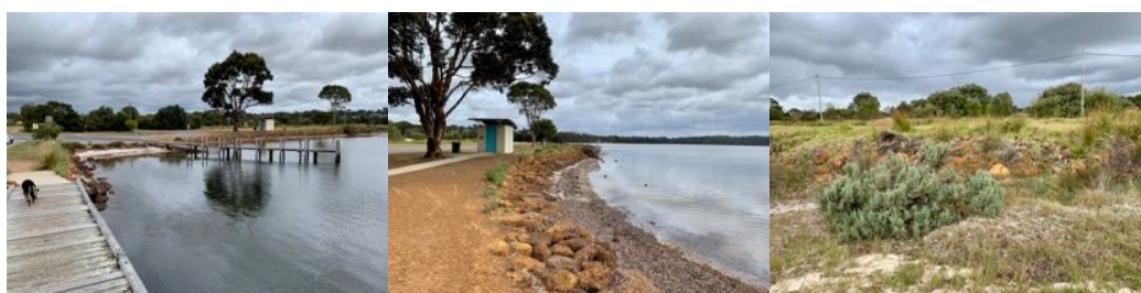
Figure 5.2 Central Foreshore including boat ramp and jetty (left), rock revetment protecting path, toilet block, large tree and road (central) and buried rock revetment along road to north (right)
