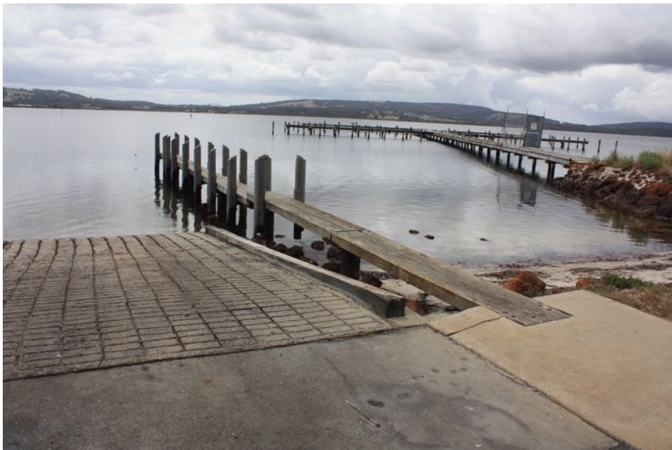
Figure 5.4 Lower King Boating Facility
