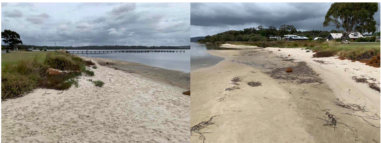
Southern termination of laterite rock revetment.
