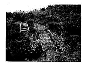
This is part of the current Circuit walk-only trail. The trail was established by Green Skills for the City several years beforehand. In April or May 2006 bikers physically removed the water bars and the short 'ladder steps' higher up the trail. Without water bars, trails such as this become drainage runnels very quickly and this is exacerbated by bike 'brake skid lines' as in the foreground of the left hand picture. In this instance the City acted quickly to repair the damage.
