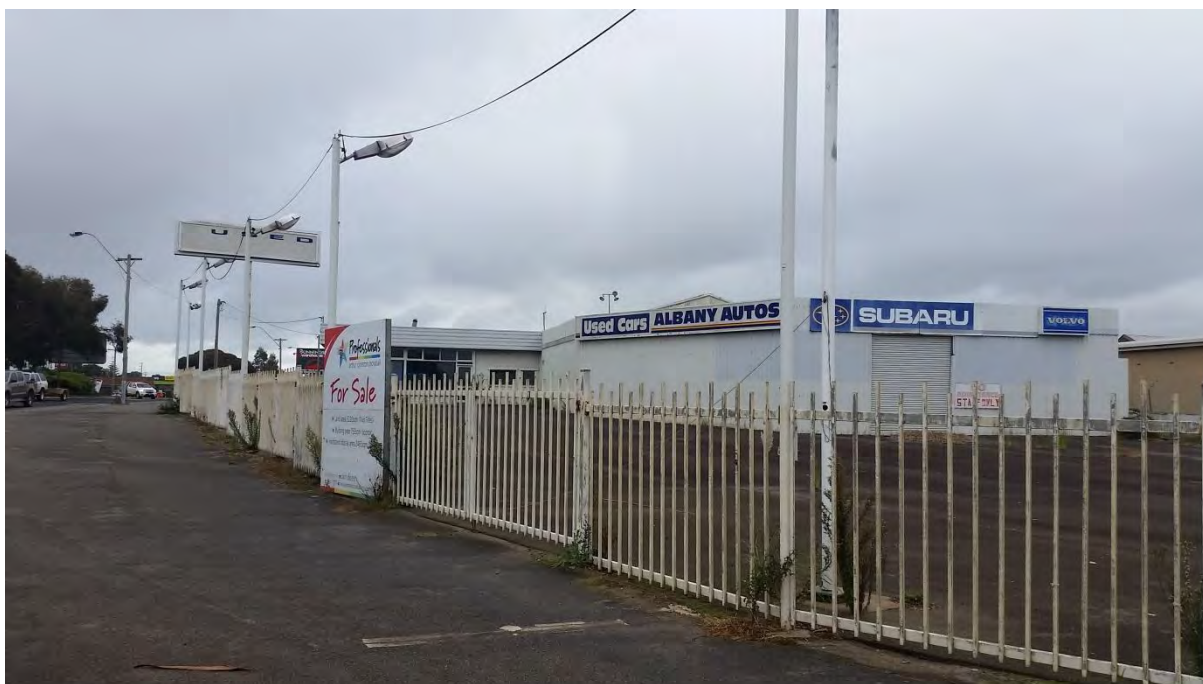
Photograph 2: Existing derelict improvements and fencing on the subject site.
