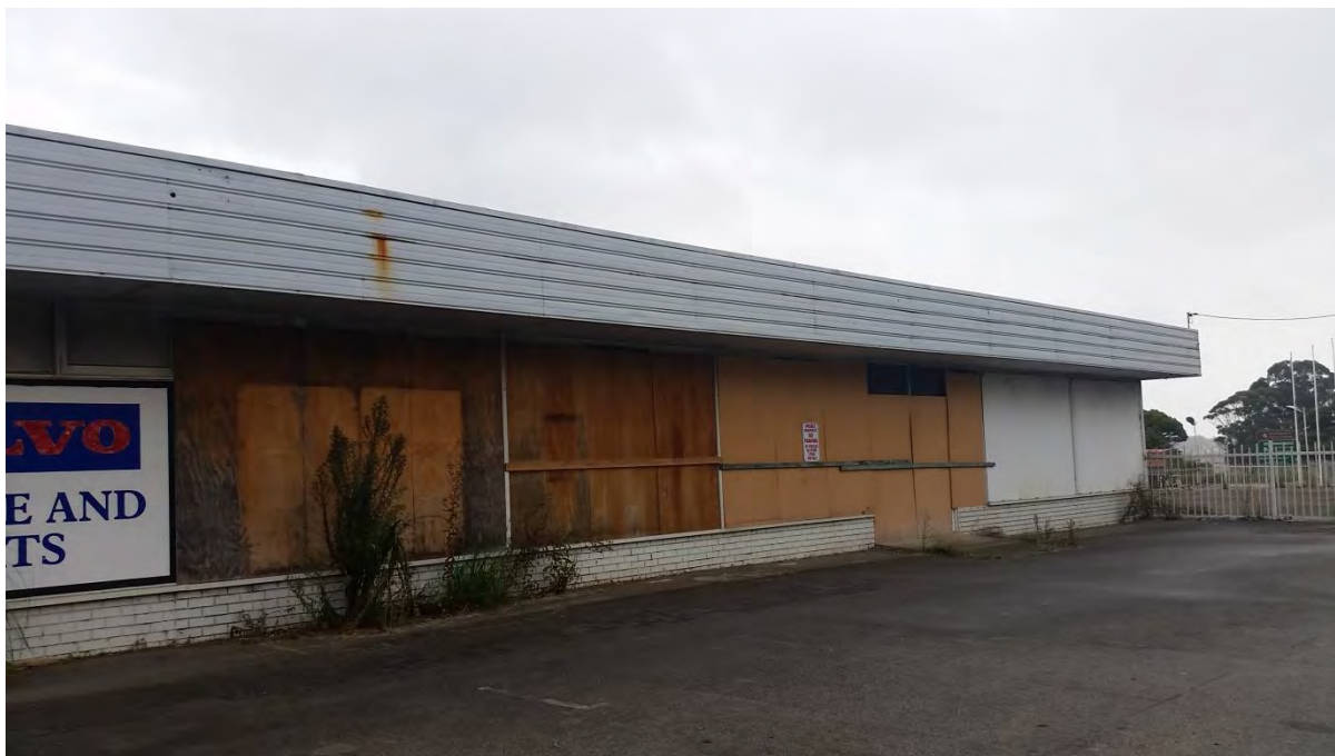
Photograph 3: Existing façade of improvements fronting Albany Highway.
