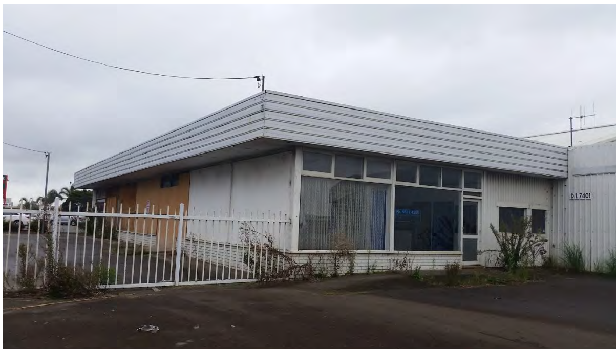
Photograph 1: Existing derelict improvements on the subject site.
