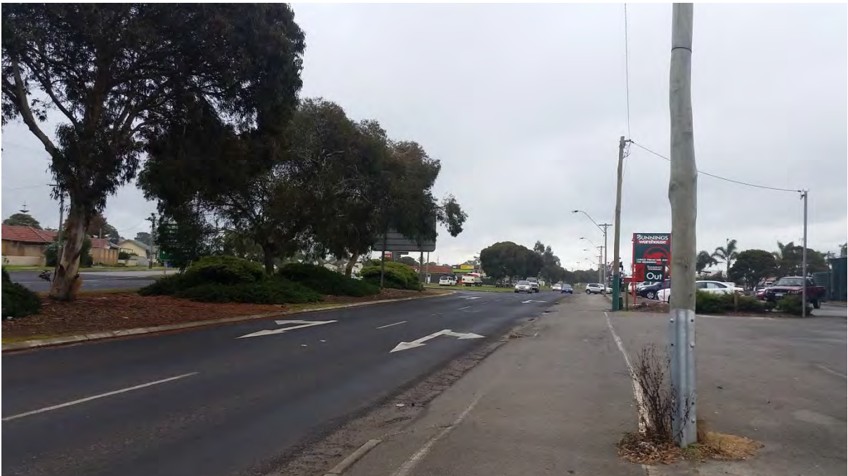
Photograph 6: View north along Albany Highway, noting existing Western Power light pole in foreground to be removed.
