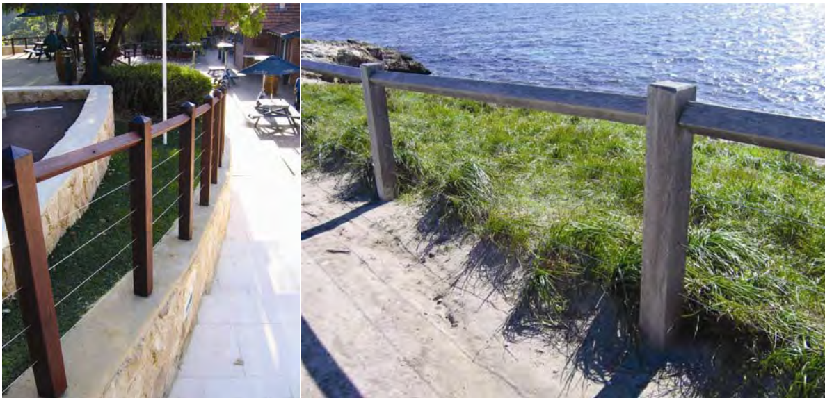
Plates 24 & 25 – Open style rural fencing will be utilised throughout the development.
