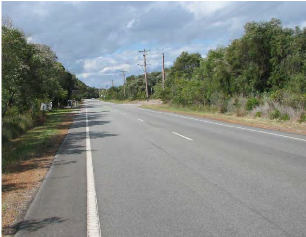
Plate 11 – Emu Point Drive near the Griffiths Street intersection
