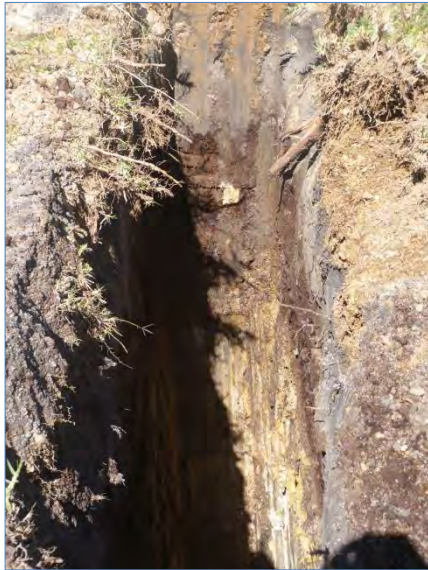
Photograph 1: Test Pit A
