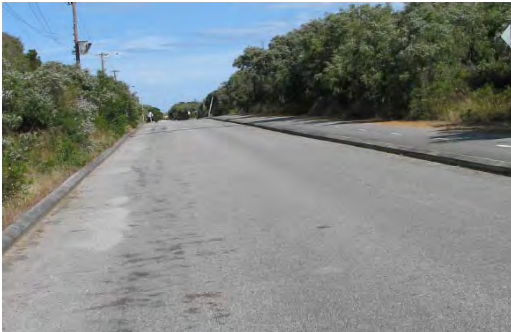
Plate 12 – Griffiths Street road pavement - looking south
