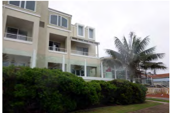
Figure 30: Middleton Beach existing housing adjacent to Barnett Street
